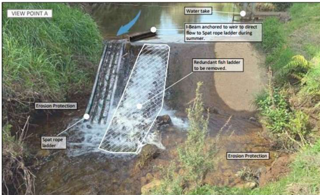
Figure 8 Proposed improvements to the Mangahewa Stream weir
