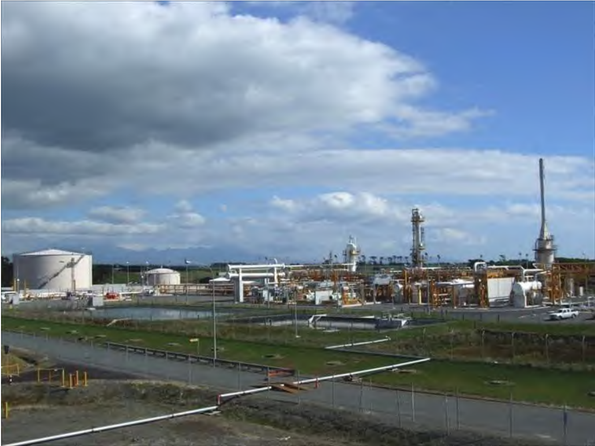
Photo 1 Pohokura Production Station
