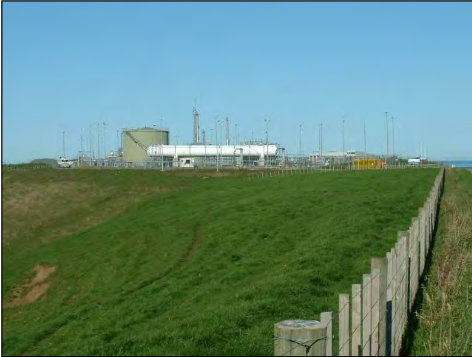
Photo 1 Rimu Production Station
