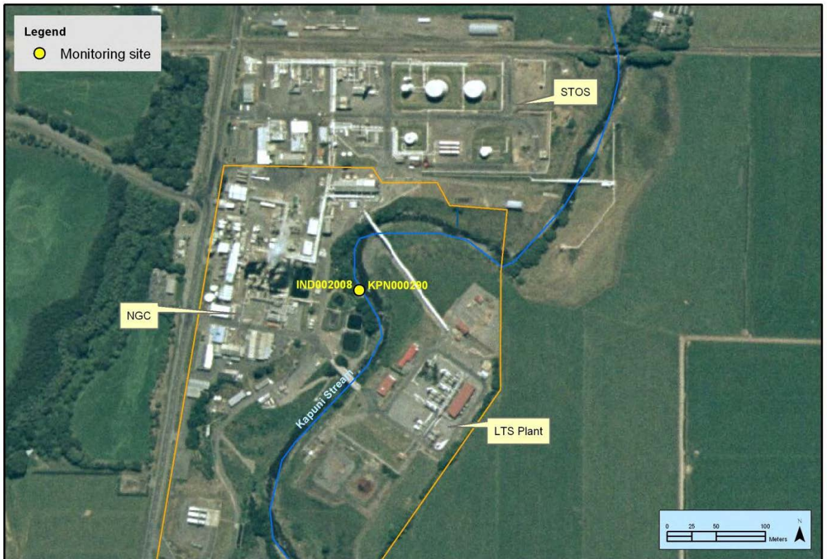
Photo 2 Vector Kapuni gas treatment plant site showing sampling locations
