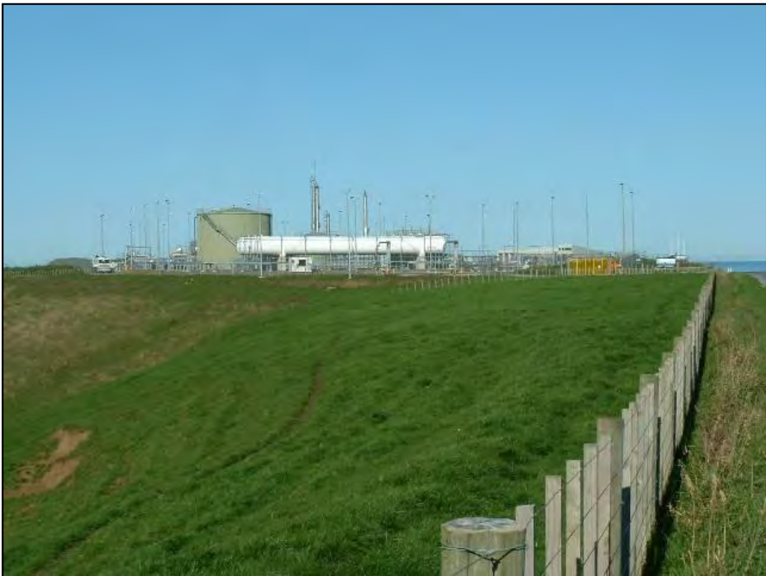
Photo 1 Rimu Production Station
