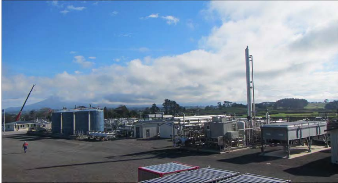
Photo 1 Cheal Production Station
