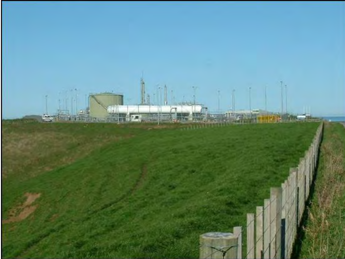
Photo 1 Rimu Production Station
