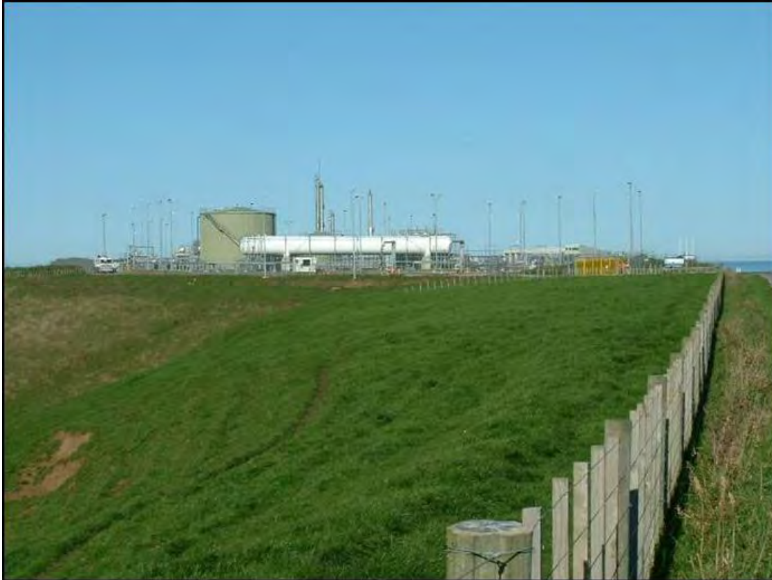
Photo 1 Rimu Production Station
