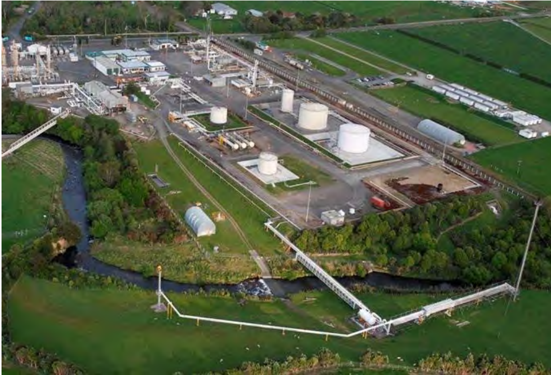
Photo 1 Kapuni Production Station
