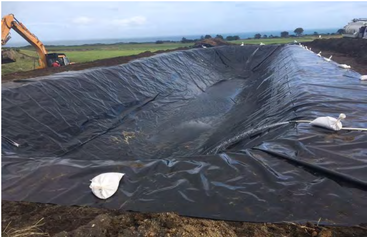
Photograph 5 Pit 1 new liner as installed
