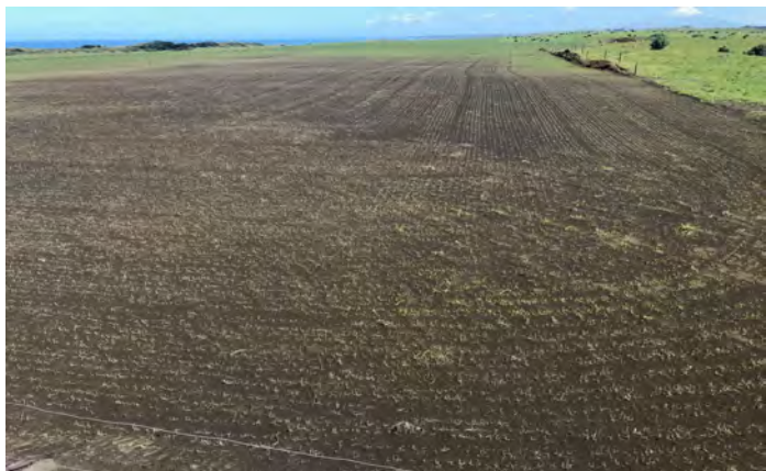
Photographs 3 and 4 Area W1911 final rehabilitation, topsoil spread, levelled and seed bed prepared and sown with oats
