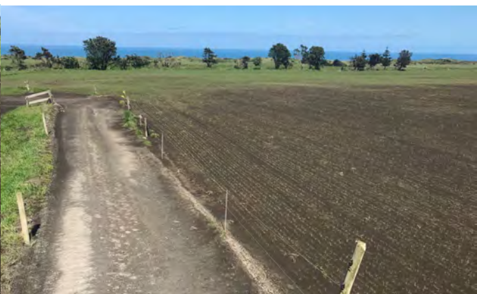
Photographs 3 and 4 Area W1911 final rehabilitation, topsoil spread, levelled and seed bed prepared and sown with oats
