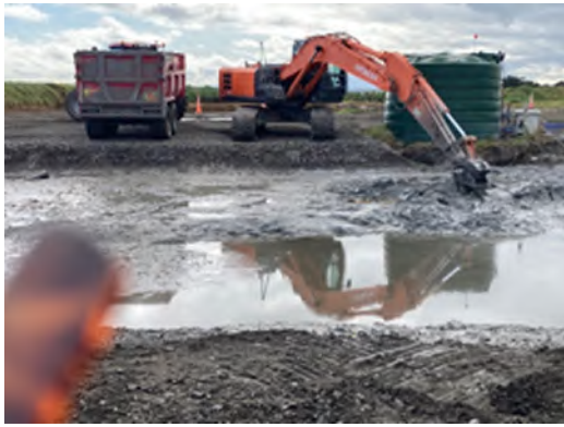
Photographs 7 and 8: 7/9/22 Recovering soil mud for spreading from Pit 1, discharging liquid mud into Pit 3 from tube
