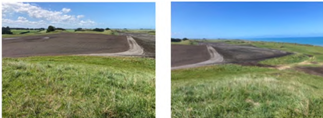
Photo 4 Top soiling completed, awaiting sowing (1/11/22) Area M2110 Stage II
