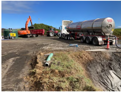
Photographs 7 and 8: 7/9/22 Recovering soil mud for spreading from Pit 1, discharging liquid mud into Pit 3 from tube
