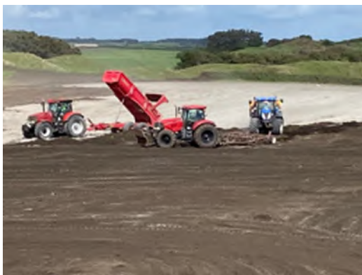
Photographs 11 and 12: 19/10/22 Topsoiling Stage 11/Phase 2 from stockpiles to the north
