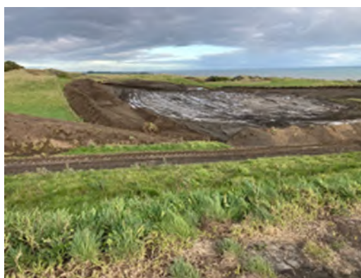
Photographs 3 and 4: 2/8/22 Formation of bunds around the spread area. Stage 11/Phase 3
