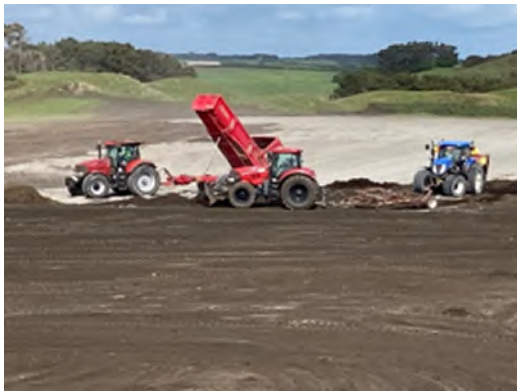
Photographs 9 and 10: 19/10/22 Topsoiling Stage 11/Phase 2 from stockpiles to the north
