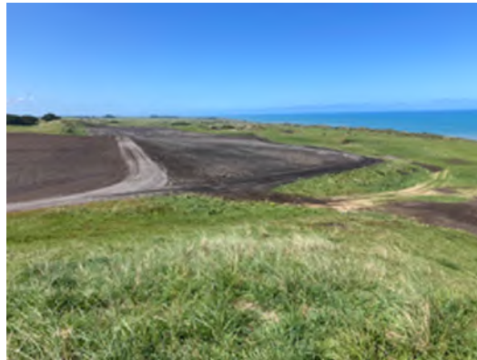
Photograph 15: 19/10/22 Topsoiling Stage 11/Phase 2 from stockpiles to the north
