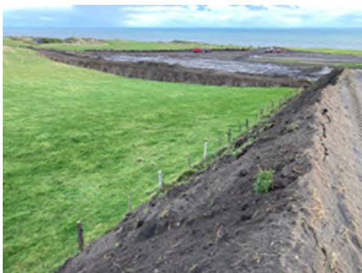
Photographs 3 and 4: 2/8/22 Formation of bunds around the spread area. Stage 11/Phase 3
