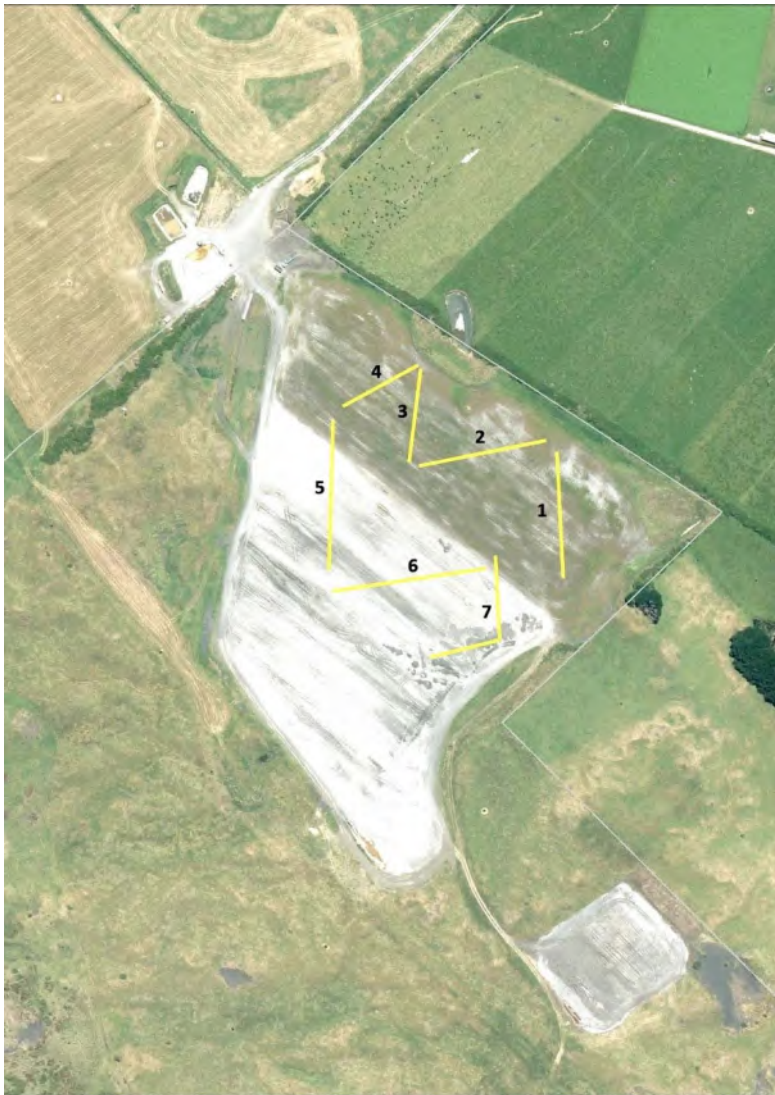
Figure 16 Location of soil transects in relation to WRS Symes Manawapou Landfarm for 2022-2023
