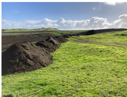
Photograph 5: Formation of bunds around the spread area. Photograph 6: Stripping Topsoil Both photos 2/8/22 - Stage 11/Phase 3
