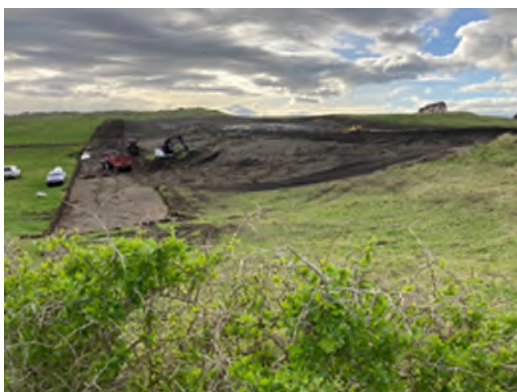
Photograph 5: Formation of bunds around the spread area. Photograph 6: Stripping Topsoil Both photos 2/8/22 - Stage 11/Phase 3
