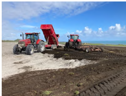
Photographs 13 and 14: 19/10/22 Topsoiling Stage 11/Phase 2 from stockpiles to the north
