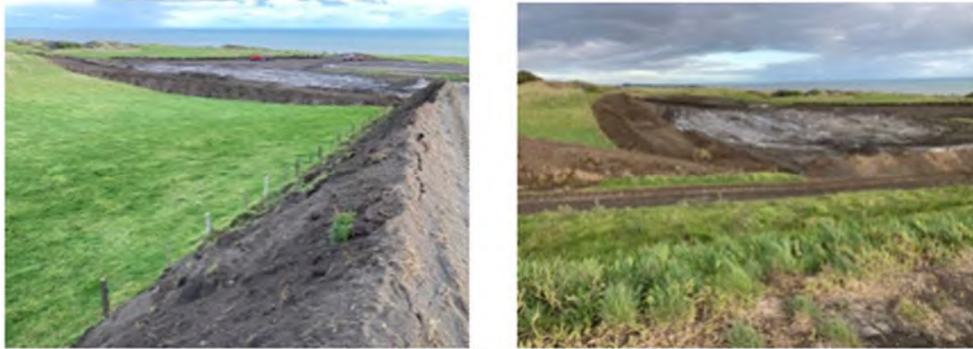
Photo 5 Formation of bunds around the spread area, Stage II/Phase 3 2/8/22
