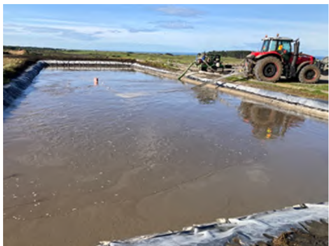
Photograph 12: 16/8/22 Pit 3 stirring, pumping, spreading
