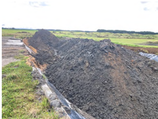
Photograph 4: 10/3/23 Pit 1 dewatered mud
