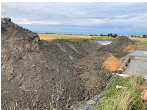
Photograph 5: 10/3/23 Pit 1 dewatered mud
