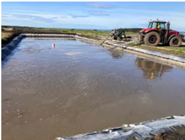
Photo 3 Pit 3 stirring and pumping
