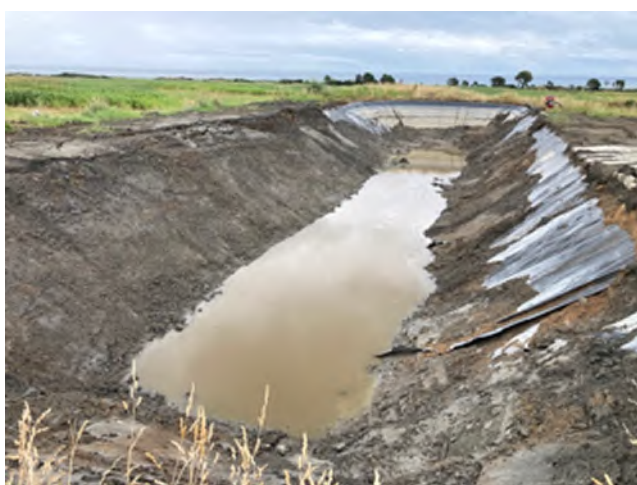
Photograph 9: 6/1/23 Pit 1 wall armouring
