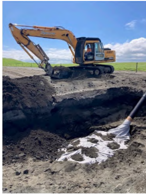
Photograph 6- Backfilling stormwater sump in sand
