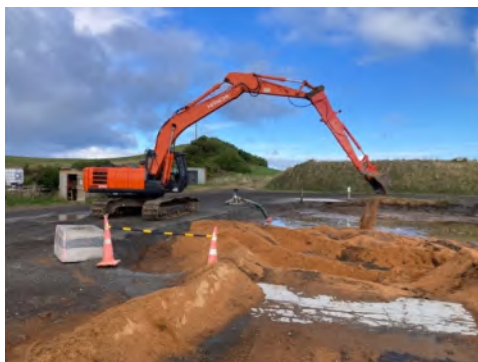
Photograph 9- Cleaning out Pit 1 with long reach digger
