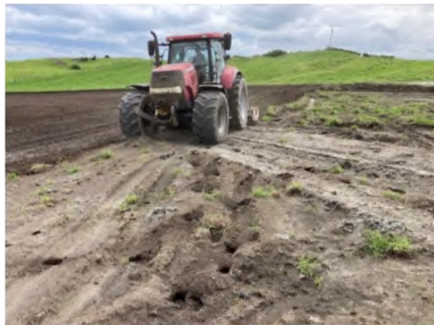
Photograph 7 – Spreading and levelling topsoil Stage2/Phase 3
