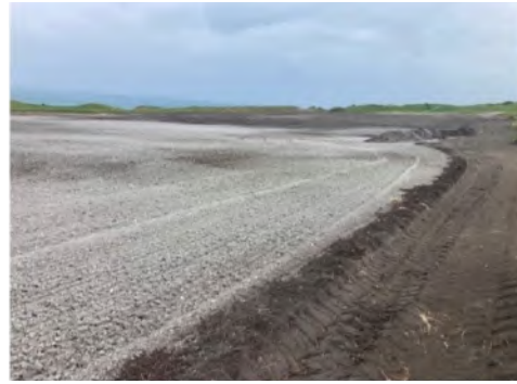
Photograph 2 -Mud drying in spread area Stage 2/Phase 3
