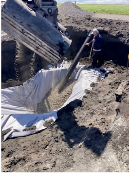
Photograph 5 – Construction of stormwater sump Stage2/Phase3
