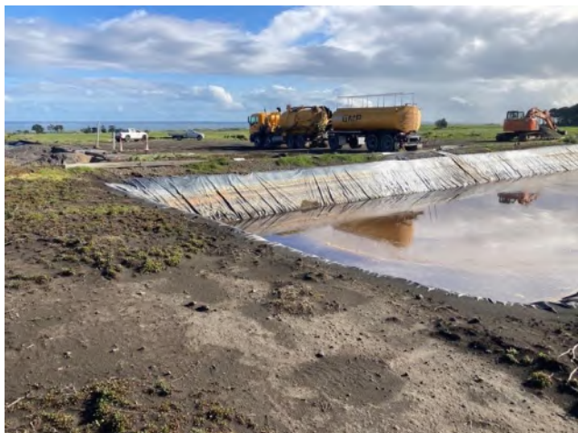
Photograph 1: 20/07/21 Waikakai GMPL Discharging Pit 3
