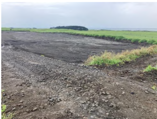
Photograph 10: 14/12/21 Waikakai Spreading Mud – Area W2205
