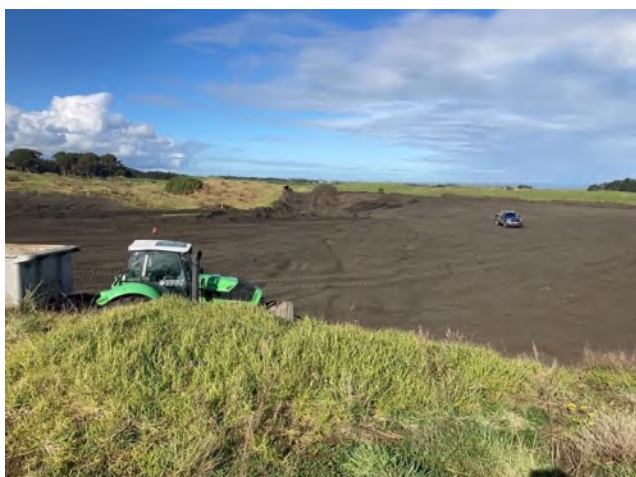
Photograph 3: 20/07/21 Waikakai Ground Preparation 2
