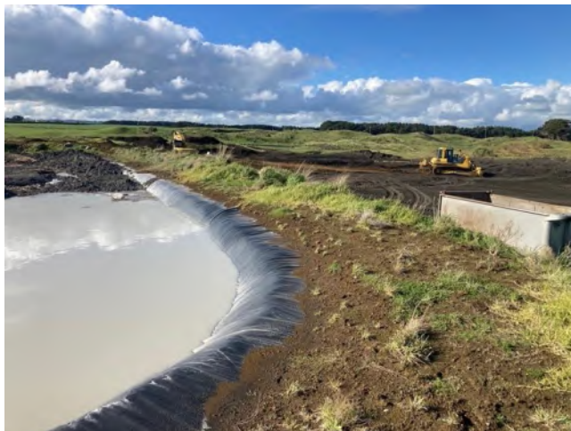
Photograph 2: 20/07/21 Waikakai Ground Preparation 1
