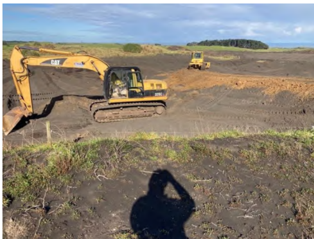
Photograph 6: 20/07/21 Waikakai Ground Preparation 3
