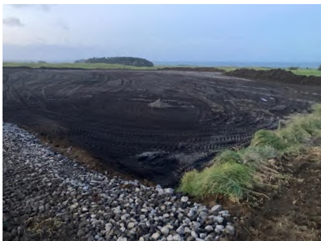
Photograph 9: 7/08/21 Waikakai Spreading Mud – Area W2205
