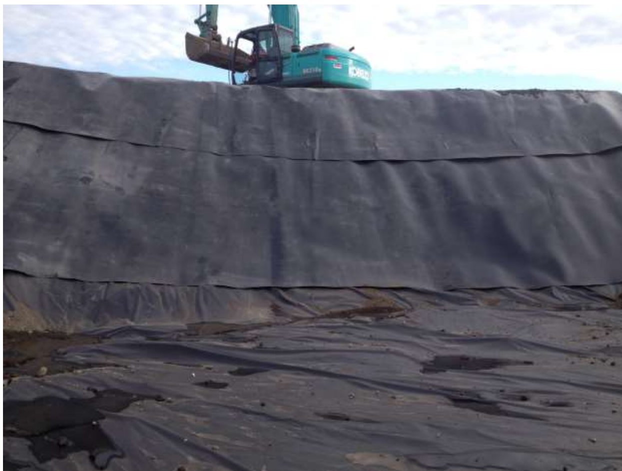
Figure 3.7 New protective liner at front of pits.
