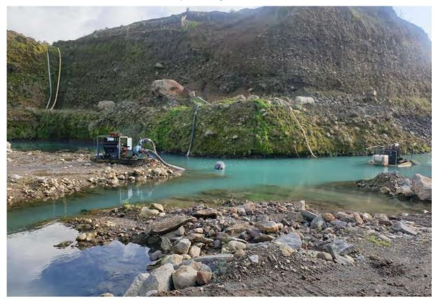
Photo 4 Ferndene Quarries Ltd groundwater seepage being pumped to the stormwater ponds, May 2019
