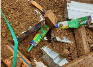
Photo 11 Unauthorised material in cleanfill including tin, wire, painted timber and Selley's packaging, June 2019
