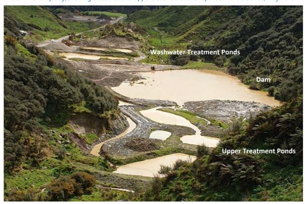
Photo 13 Uruti quarry washwater and stormwater treatment system and dam in the lower quarry site, October 2019
