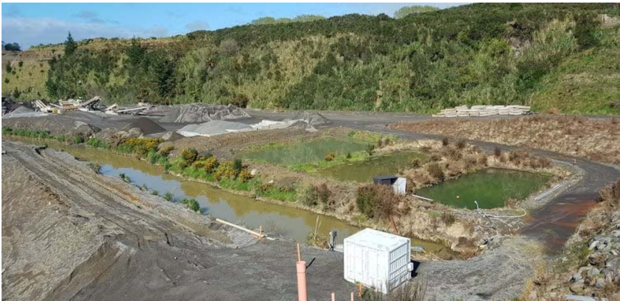
Photo 2 Washwater ponds and stormwater Pond A in the foreground, October 2021
