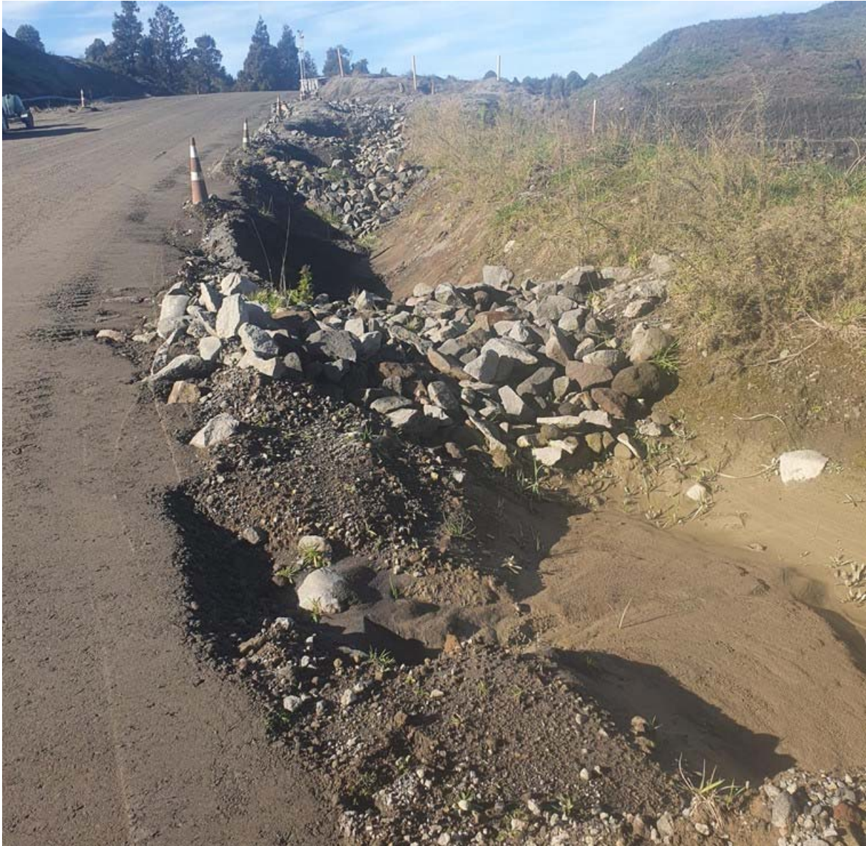
Photo 7 Site sediment control, June 2022
