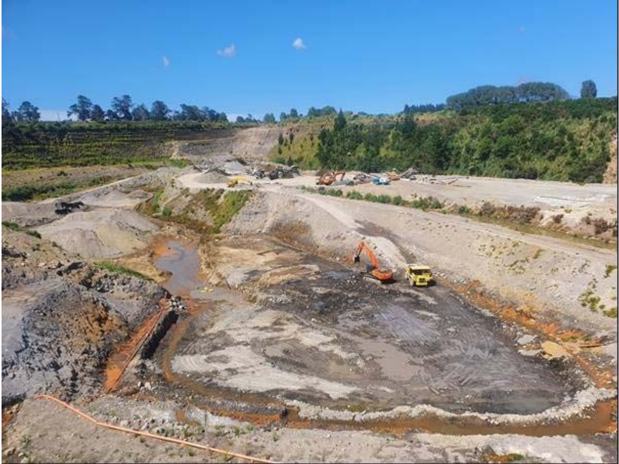
Photo 1 Excavation area west of the washwater ponds, January 2021
