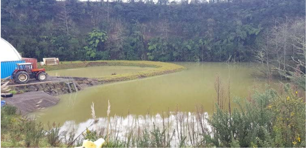
Photo 3 Stormwater Ponds B and C, July 2021
