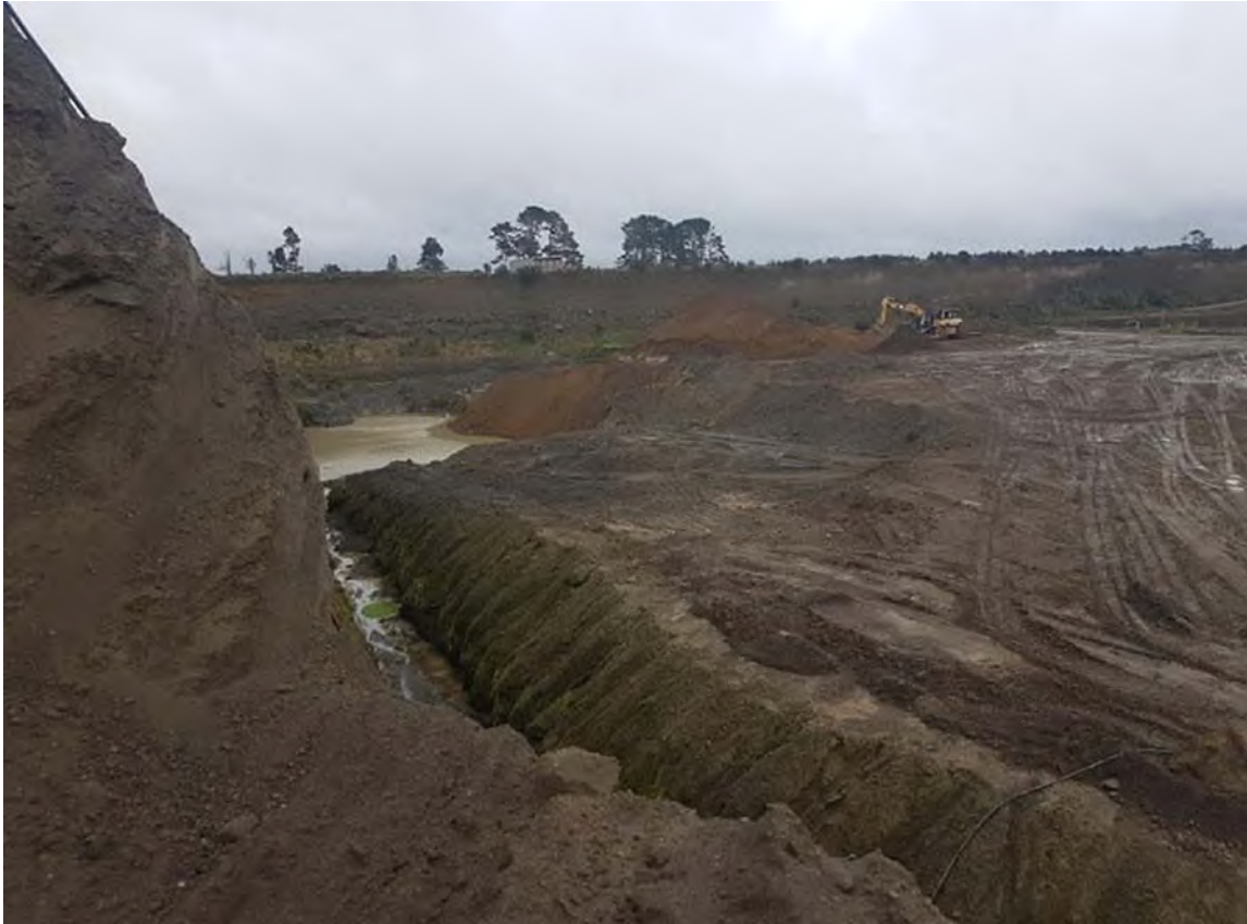
Photo 2 Burgess & Crowley East Road quarry site below the wetland, 28 May 2019
