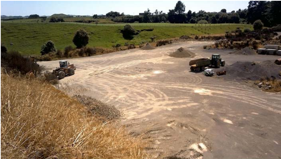
Photo 16 Taunt Contracting Ltd Bird Road quarry site 6 December 2017
