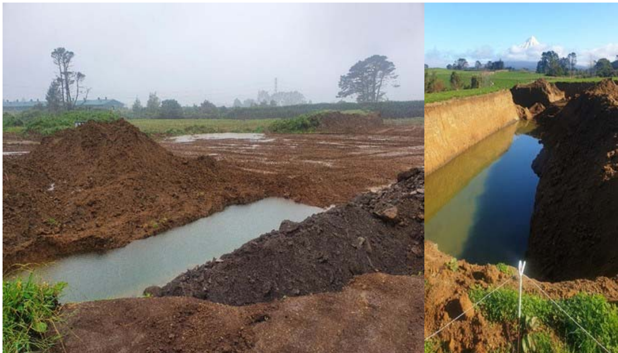
Photo 7 Hey Trust Quarry settling pond as of December 2021 (left) discharging to Kahouri Stream and/or the unnamed tributary. Settling pond (right) looking toward open ring drain system
