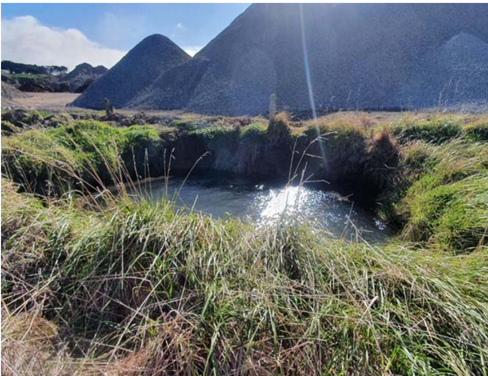
Photo 11 Settling pond 2 May 2022
