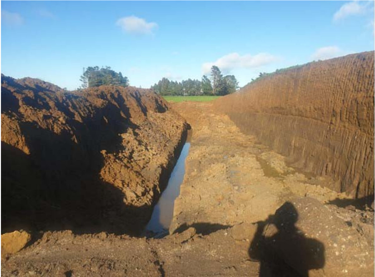
Photo 8 The majority of the site is directed through open drains to one of two settling ponds. Discharge then to Kahouri Stream and/or the unnamed tributary. Photo captured 23 June 2021
