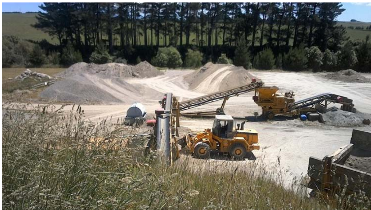
Photo 6 DM & DL Bourke Onewhaia Road quarry site 6 December 2017
