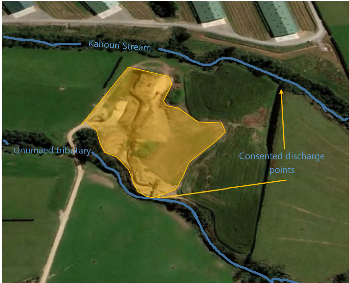
Figure 6 Hey Trust Monmouth Road quarry site footprint as of May 2022 (Google Earth)
