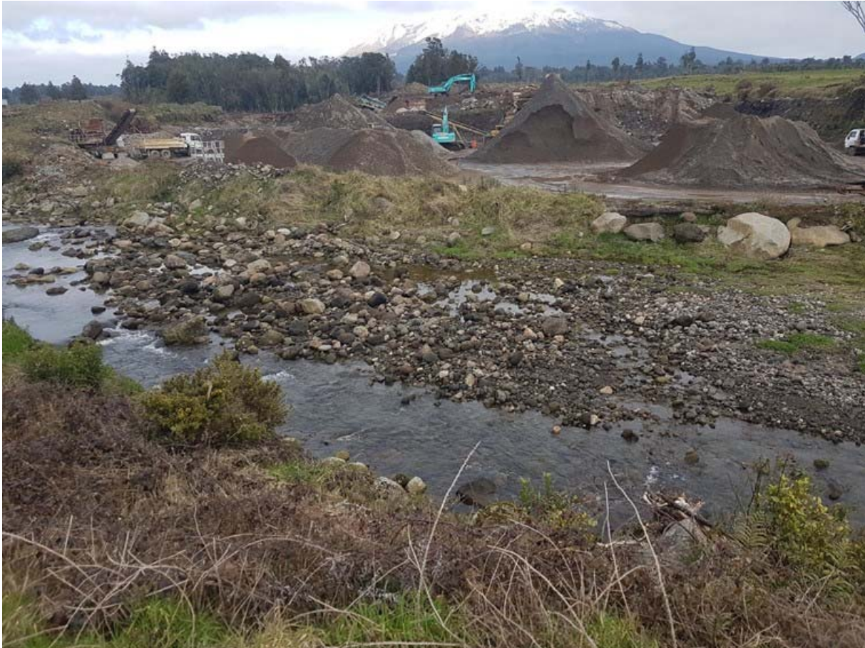
Photo 1 Bunn Earthmoving Ltd Surrey Road quarry site 7 July 2019
