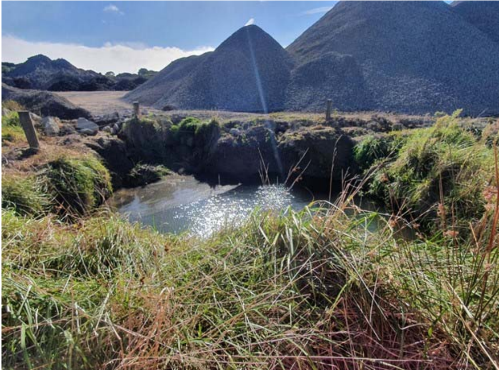
Photo 10 Settling pond 1 May 2022
