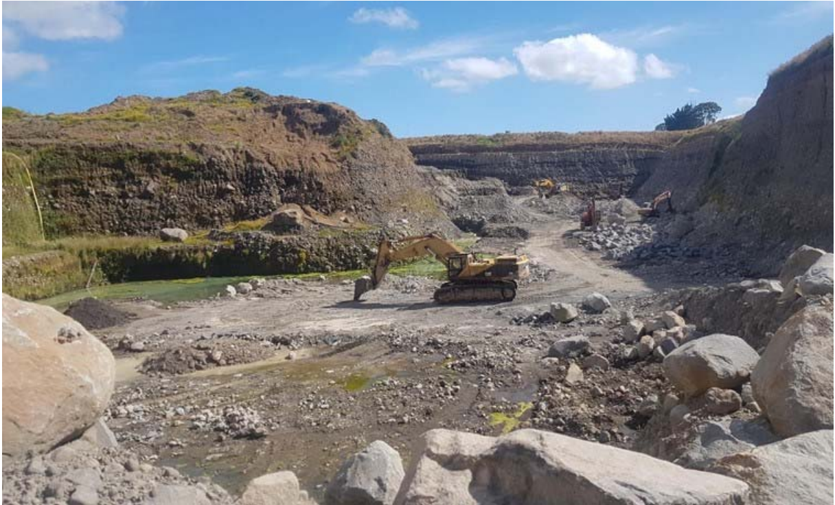
Photo 8 Ferndene Quarries Ltd excavation pit, January 2019
