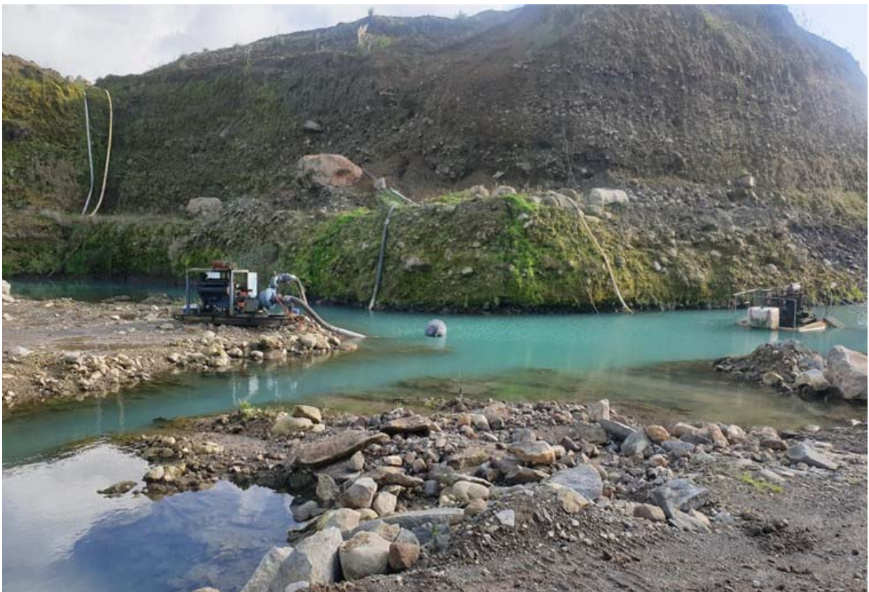
Photo 9 Ferndene Quarries Ltd groundwater seepage being pumped to the stormwater ponds, May 2019
