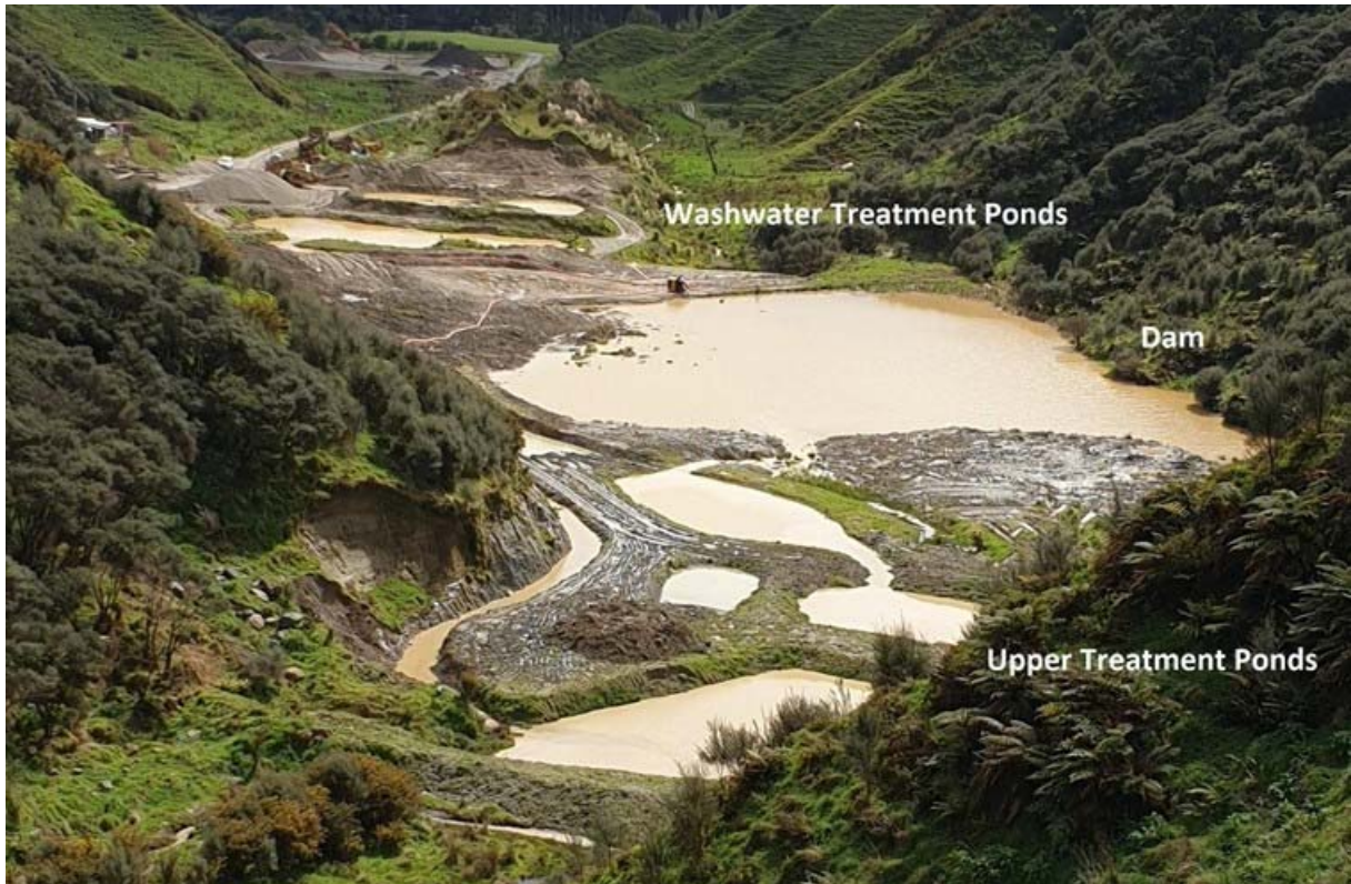
Photo 23 Uruti quarry washwater and stormwater treatment system and dam in the lower quarry site, October 2019
