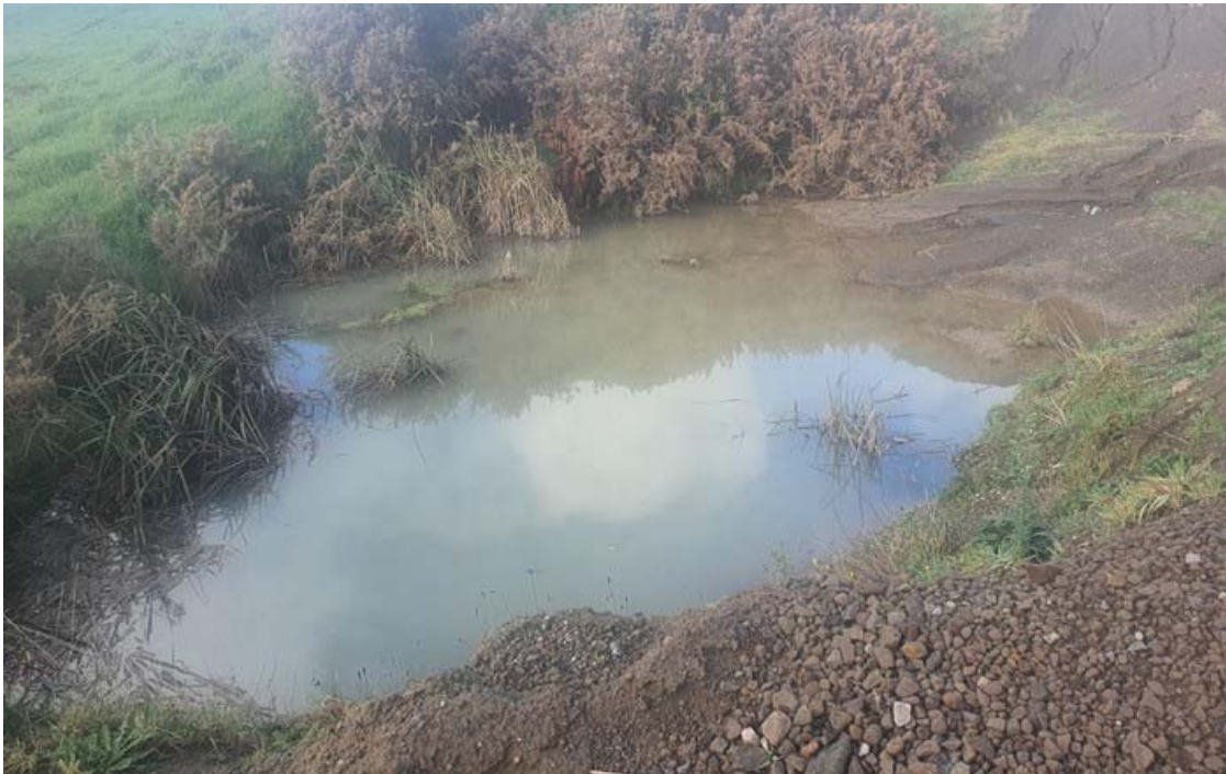
Photo 6 Jones Quarry Ltd quarry settlement pond May 2022
