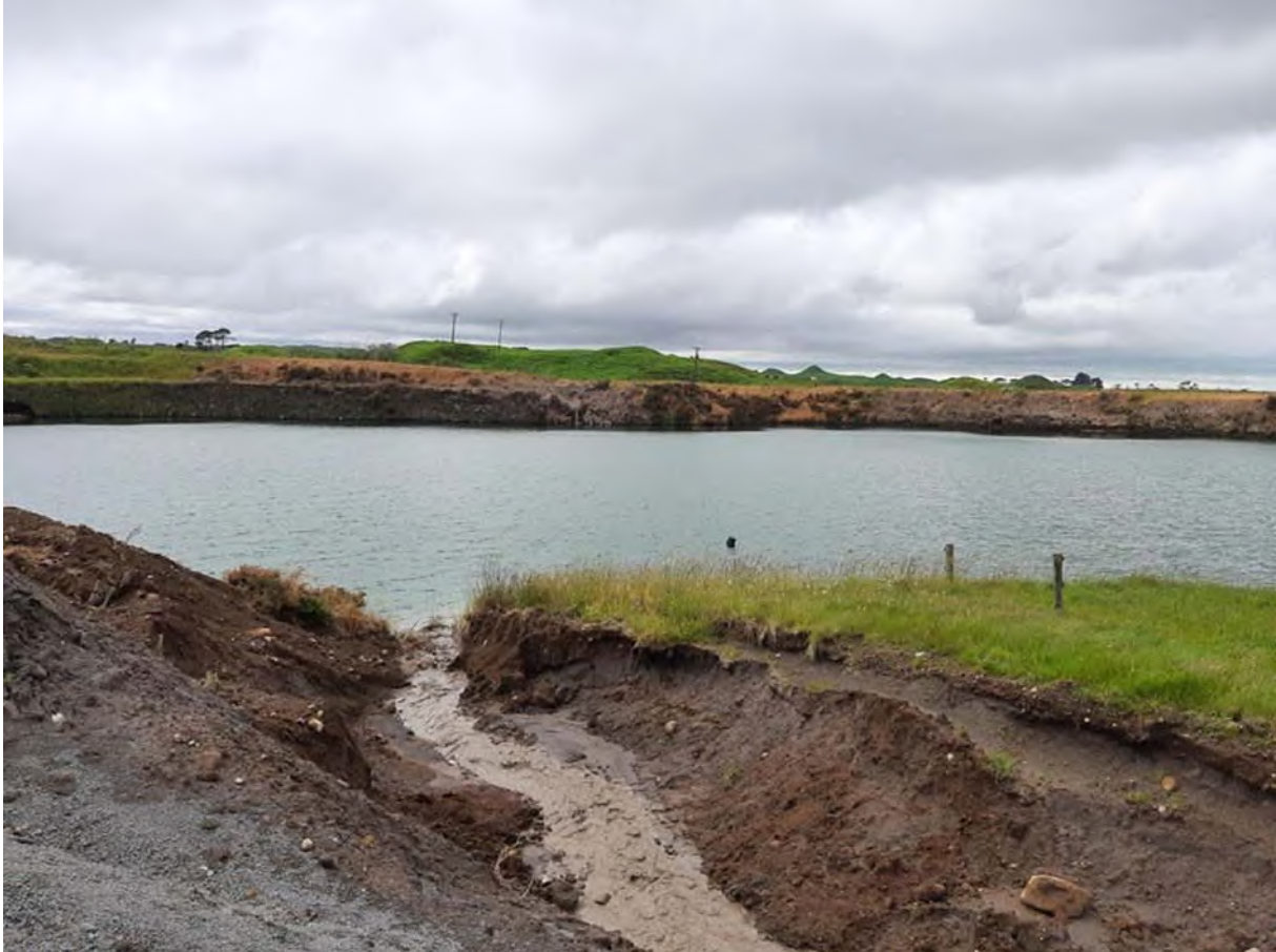
Photo 32 Wiremu Road Quarry, washwater discharge point to main lake, December 2021
