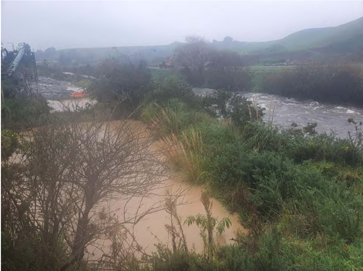
Photo 30 Whitaker Civil Engineering Ltd quarry, settlement pond and clean river, May 2022
