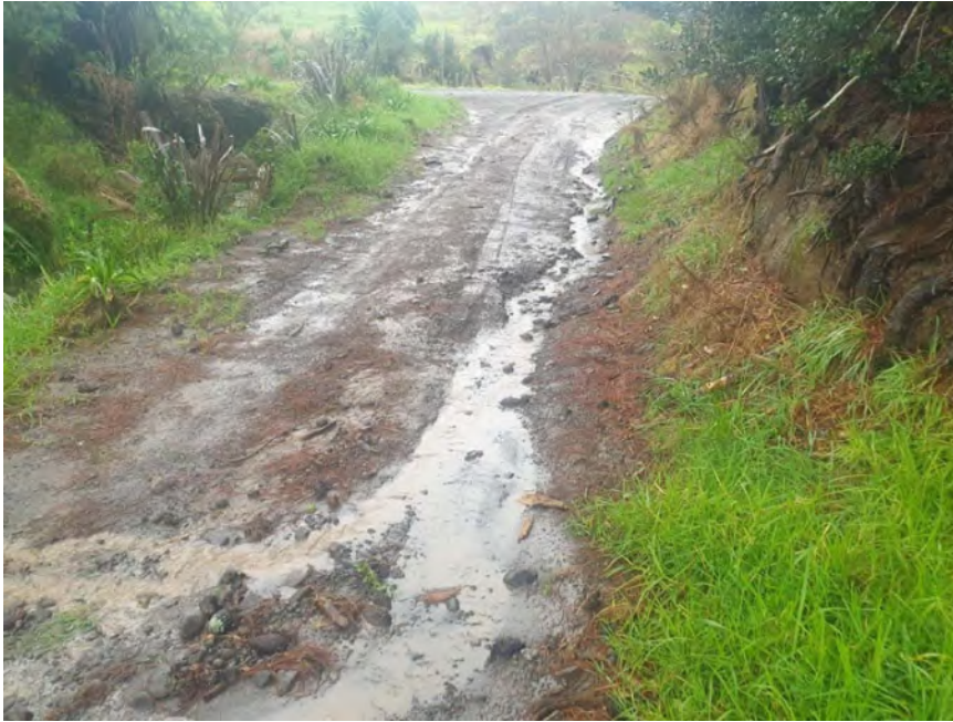
Photo 27 R J Dreaver quarry, stormwater bypassing the treatment system, June 2021
