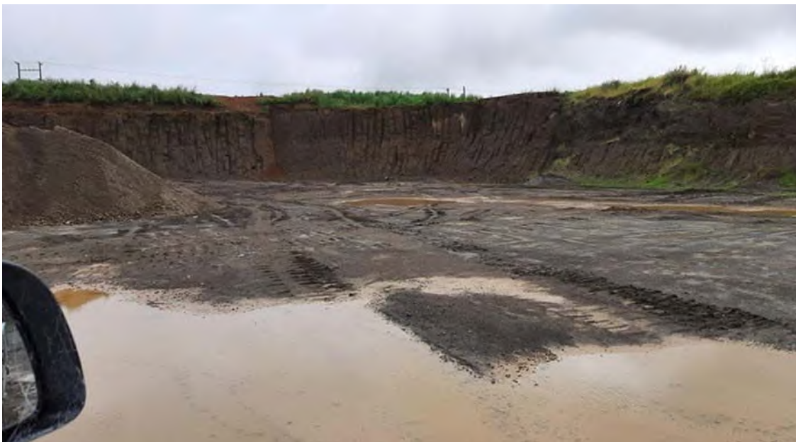
Photo 2 AA Contracting Ltd quarry excavation area December 2021
