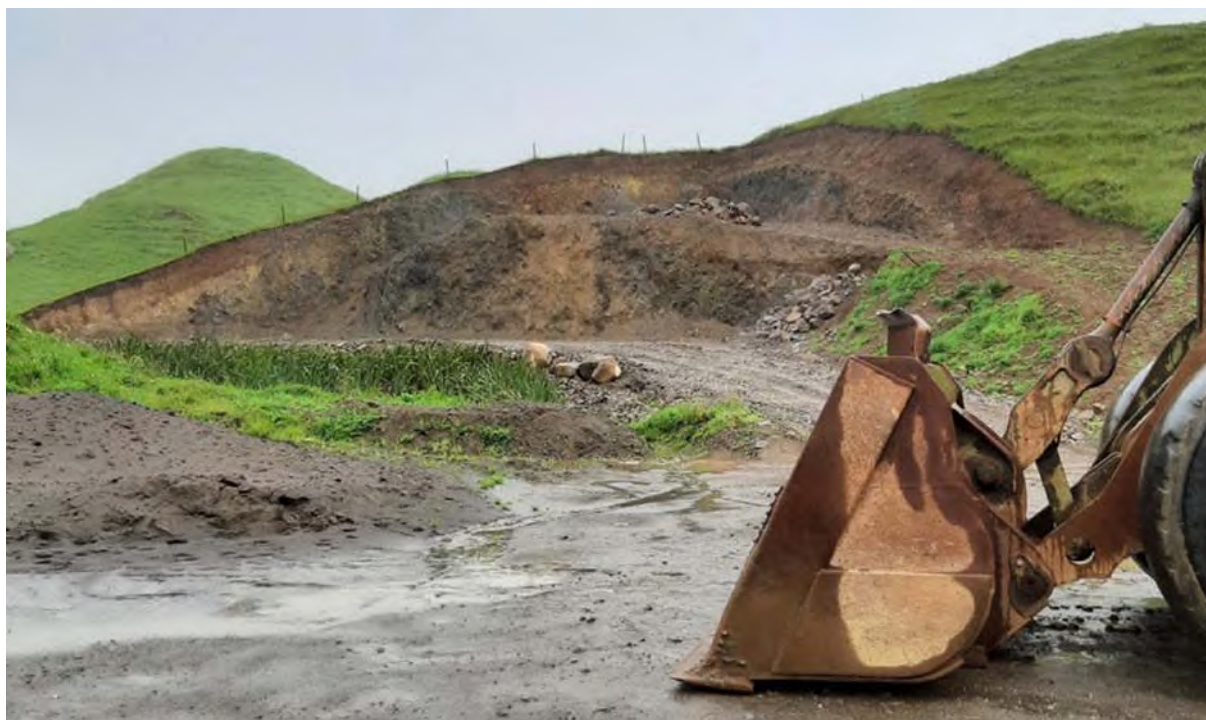
Photo 18 Goodin AG Ltd quarry site, new excavation area, December 2021
