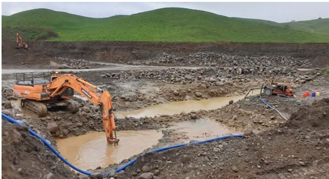
Photo 19 Hydro Road quarry construction of new settlement ponds, July 2019
