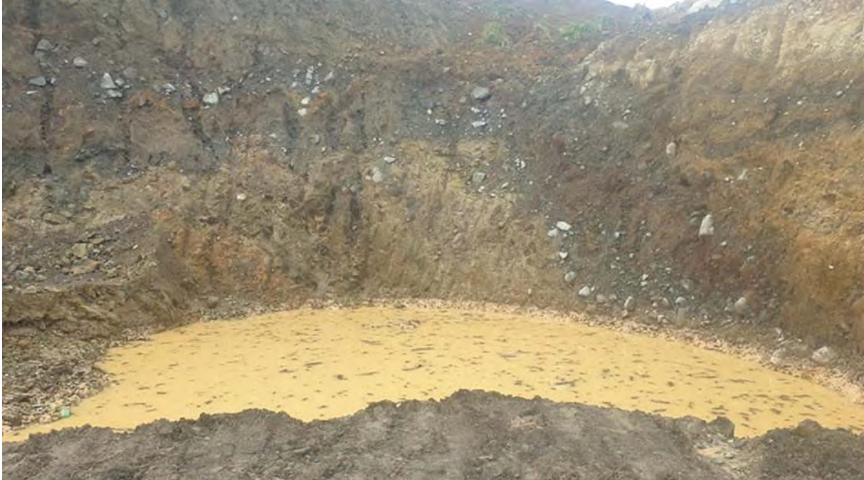
Photo 16 Puniho Road quarry new soak hole, June 2021
