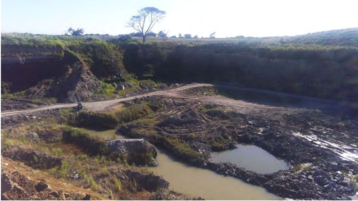
Photo 14 GR and LJ Jones quarry in Waitara
