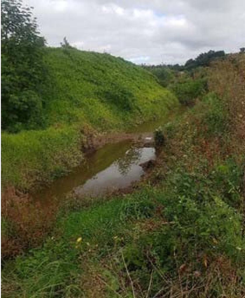
Photo 26 Stormwater pond, May 2019
