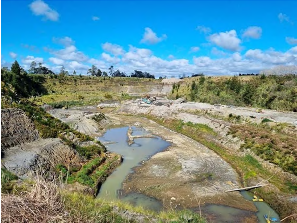
Photo 1 Excavation area west of Pond A, September 2023
