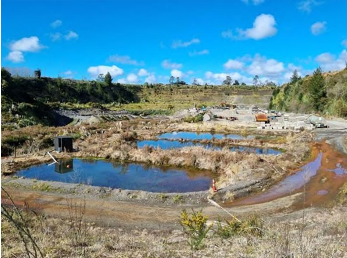
Photo 3 Ponds A1 to A3 are used to capture stormwater as aggregate is no longer washed on site
