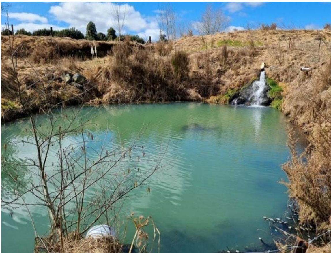
Photo 6 Pond E, the second of the gravity fed stormwater ponds, September 2023
