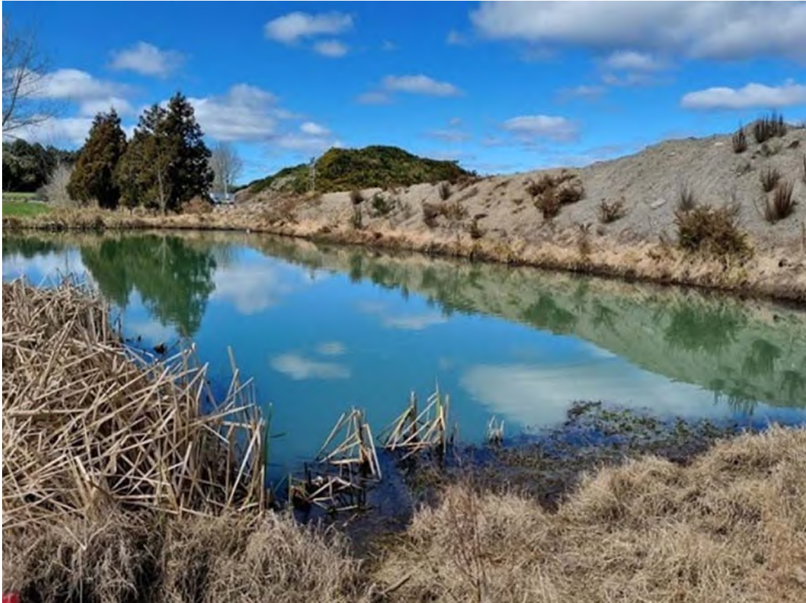
Photo 5 Pond D, the first of the gravity fed stormwater ponds, September 2023
