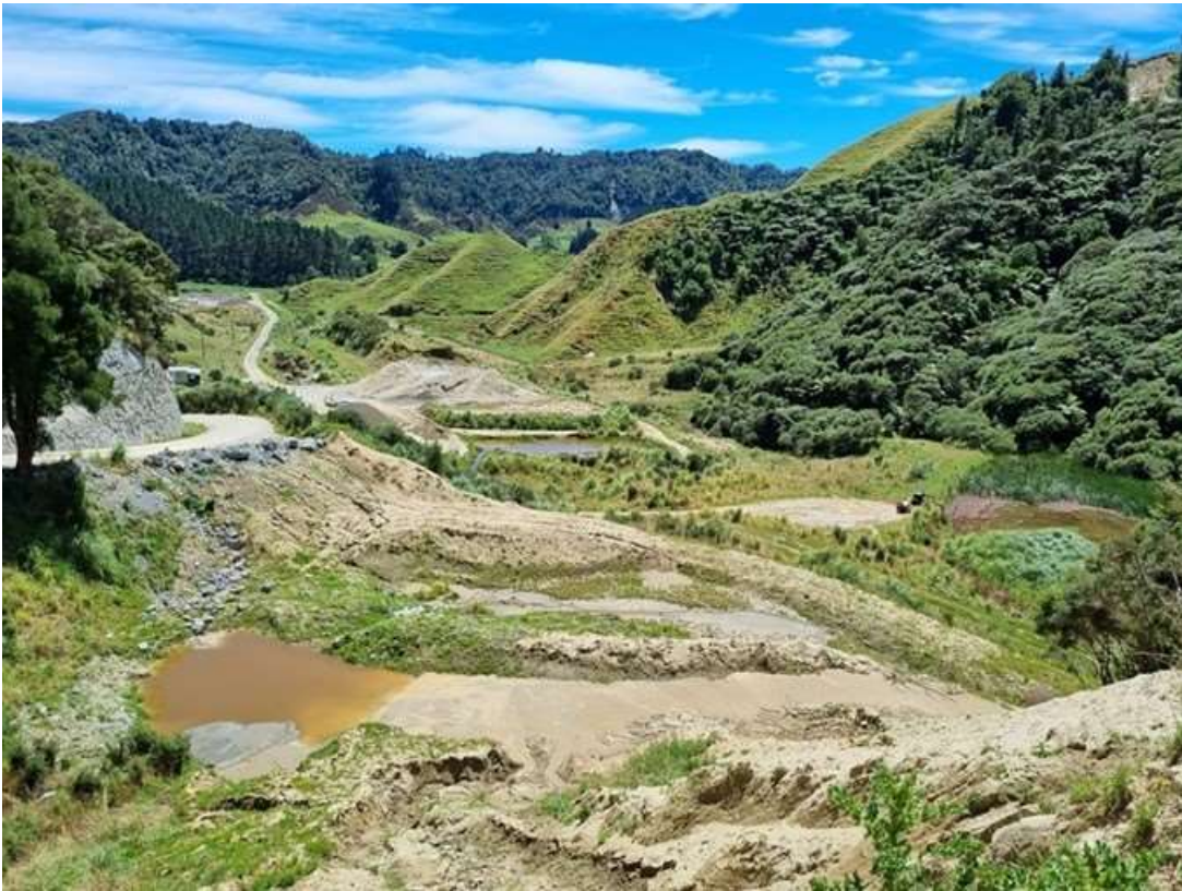
Photo 15 Looking down towards the wash plant and central laydown area, 30 January 2024
