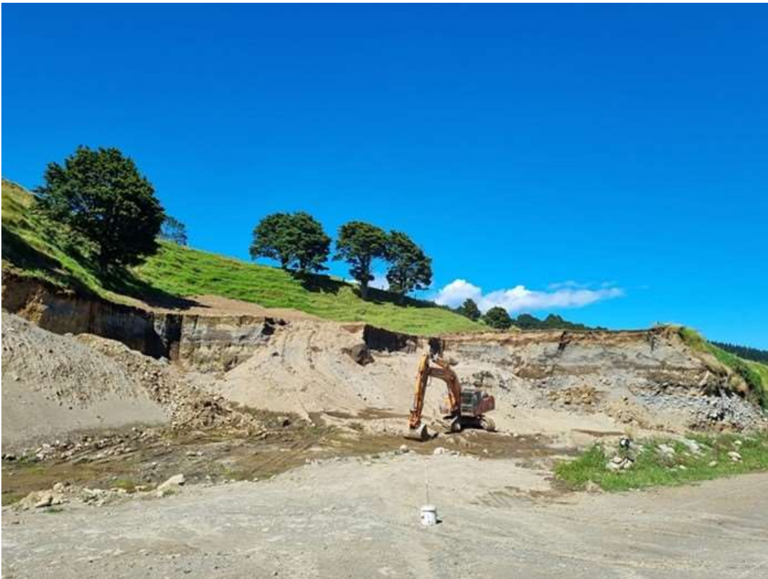
Photo 13 New excavation area, 30 January 2024
