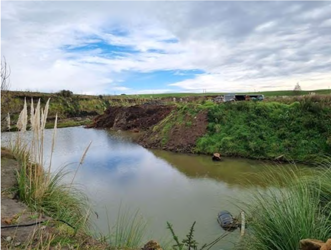
Photo 1 Former stormwater pond into which cleanfill material is discharged as part of the site rehabilitation plan
