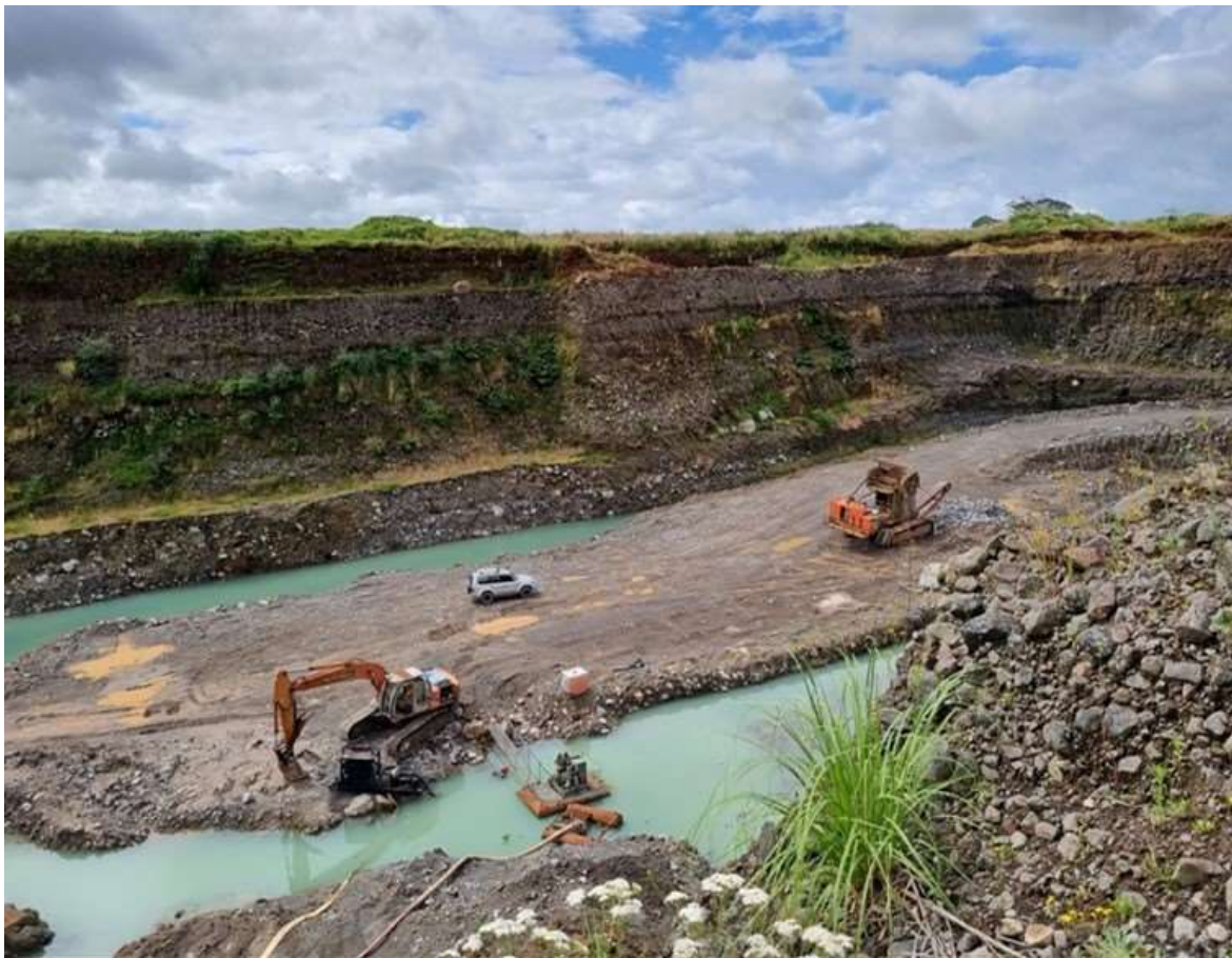
Photo 5 Main excavation pit
