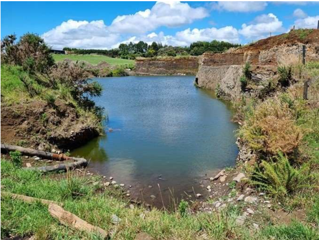
Photo 21 Sediment retention pond on the western margin of the quarry site
