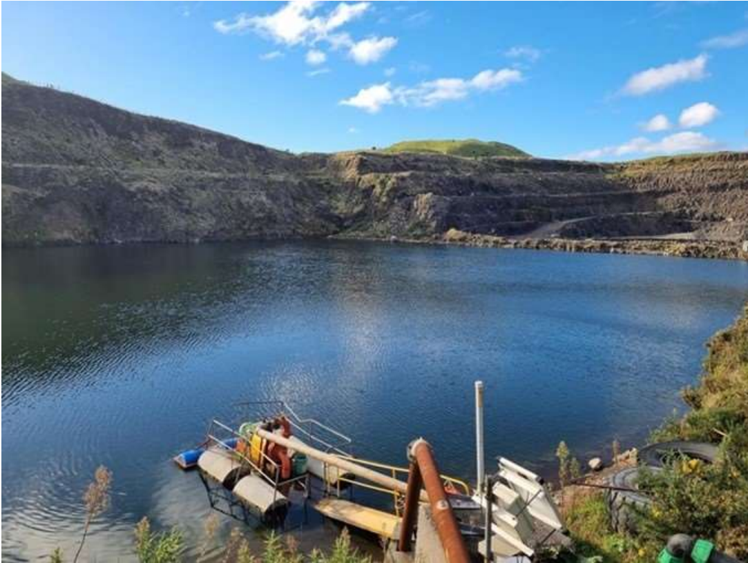
Photo 26 Settlement pond, upper site
