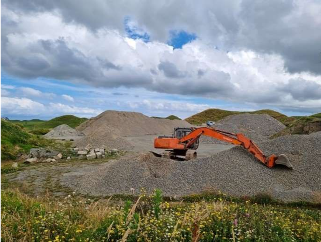
Photo 10 GoodinAg Quarry laydown area, 22 January 2024
