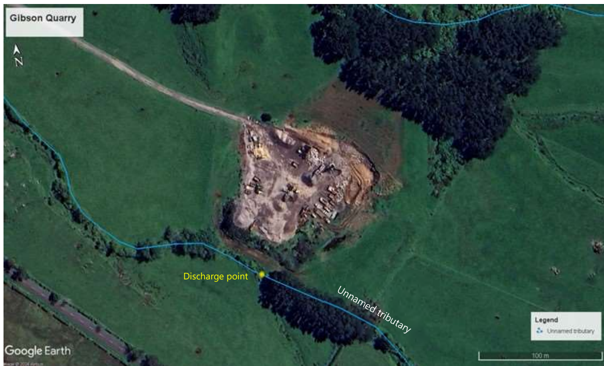
Figure 8 Gibson Family Trust Puniho Road quarry site
