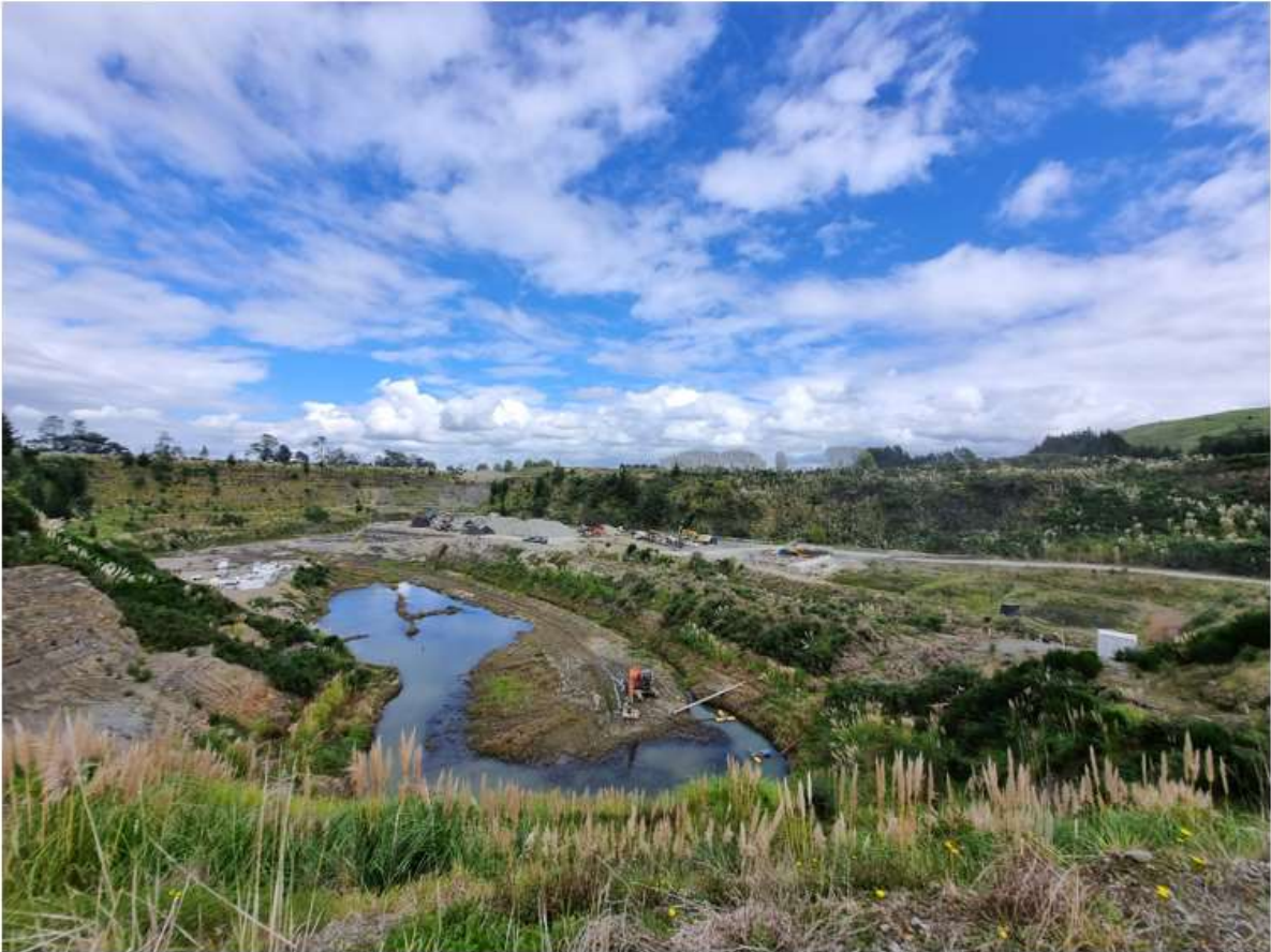
Photo 1 Excavation pit west of Pond A
