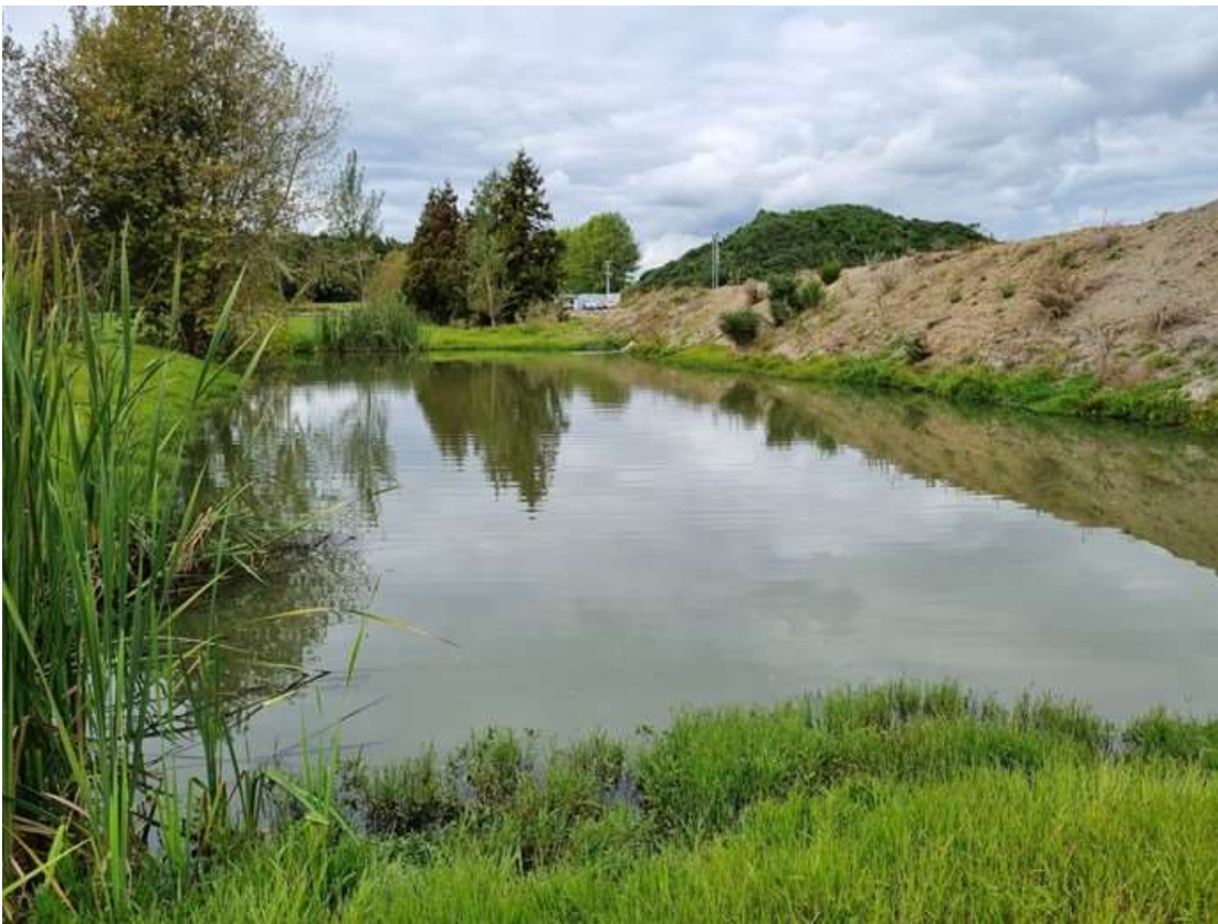
Photo 4 Pond D, the first of the gravity fed stormwater ponds, April 2024
