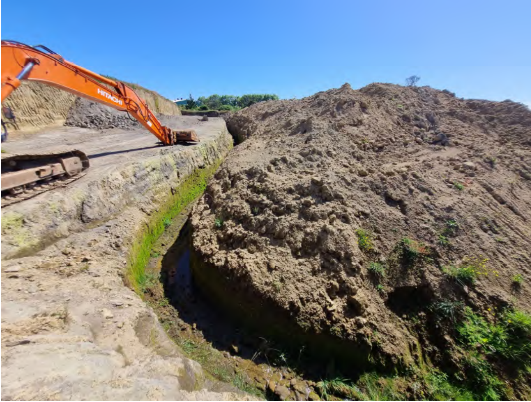
Photo 7 The majority of the site is directed through open drains to one of two settling ponds. Discharge then to Kahouri Stream and/or the unnamed tributary (25 January 2024)
