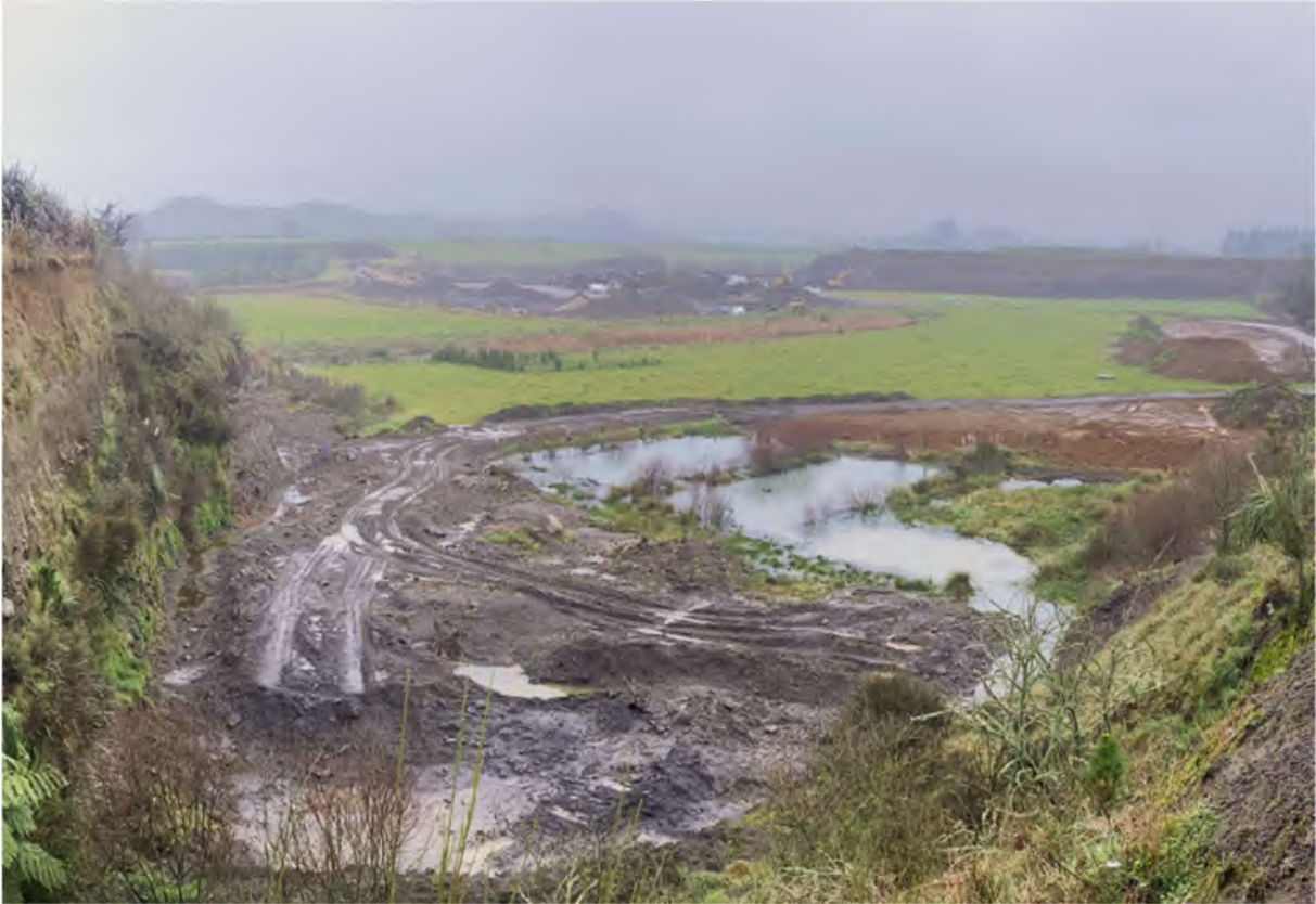
Photo 2 Burgess & Crowley East Road quarry site as at 29 June 2022
