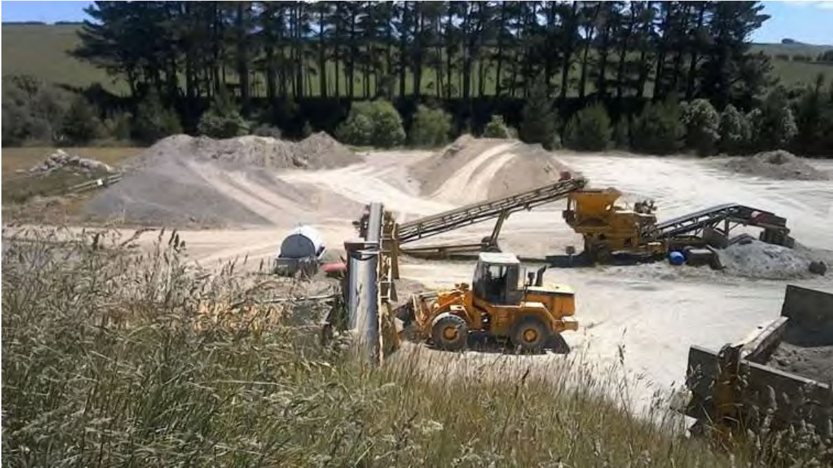
Photo 5 DM & DL Bourke Onewhaia Road quarry site 6 December 2017
