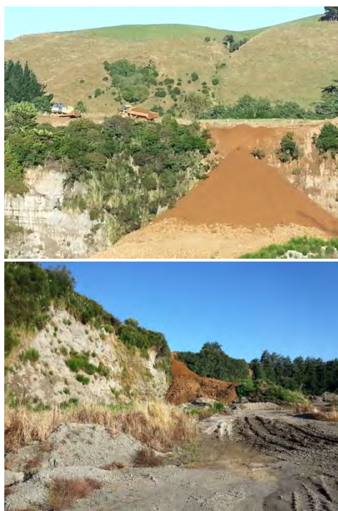
Photos 1 & 2 Recent progress with re- instatement, February, 2015
