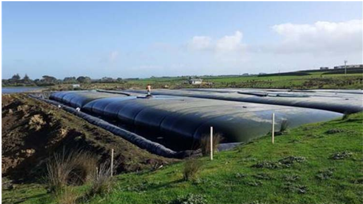
Photo 3 Geotextile bags at 840 tDS in September 2020
