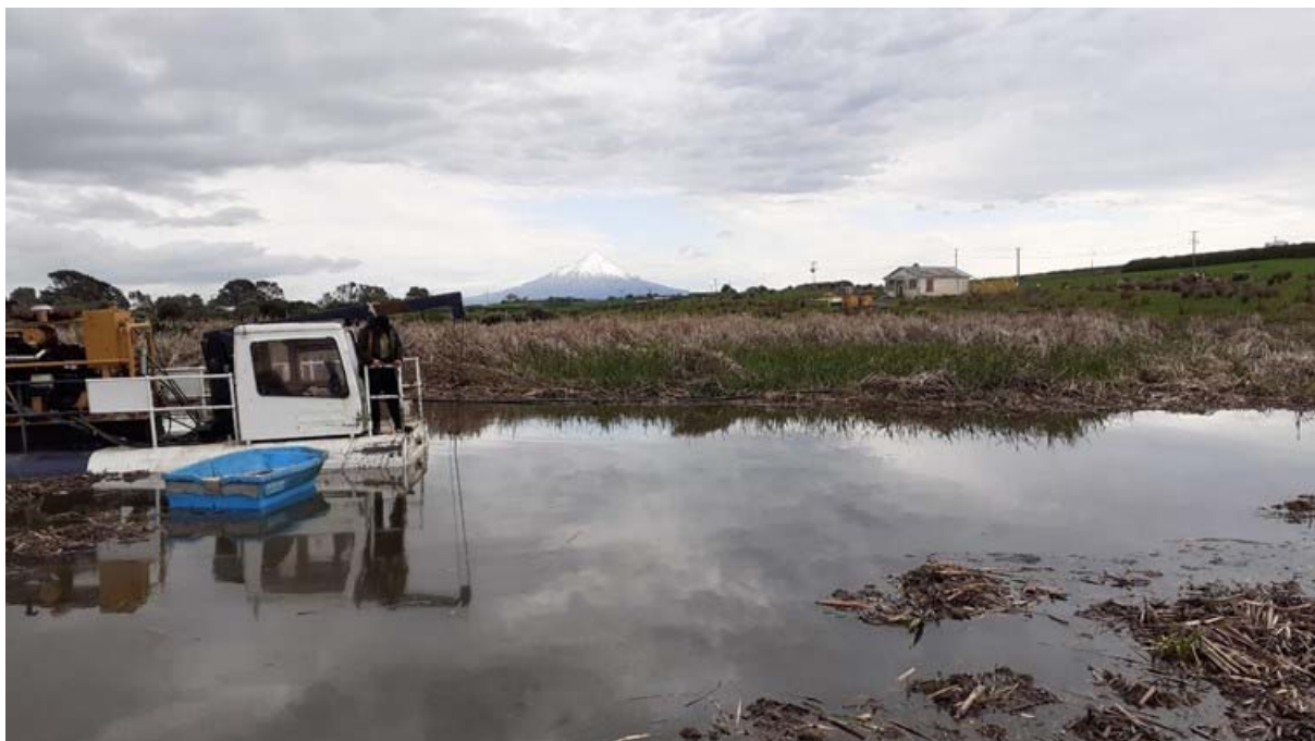
Photo 2 Desludging of the anaerobic lagoon
