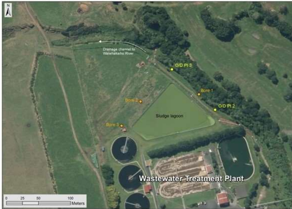
Figure 2 NPWWTP sludge lagoon and groundwater bore and drain sampling sites
