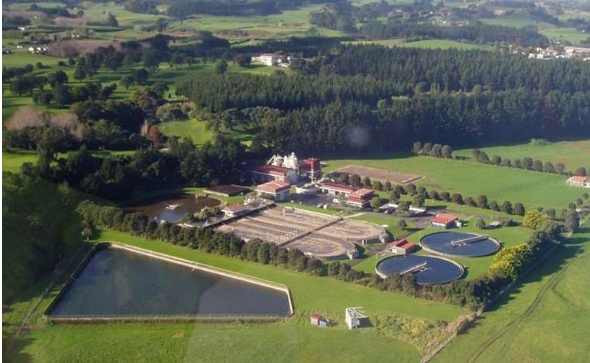
Photo 1 The New Plymouth Wastewater Treatment Plant prior to expansion
