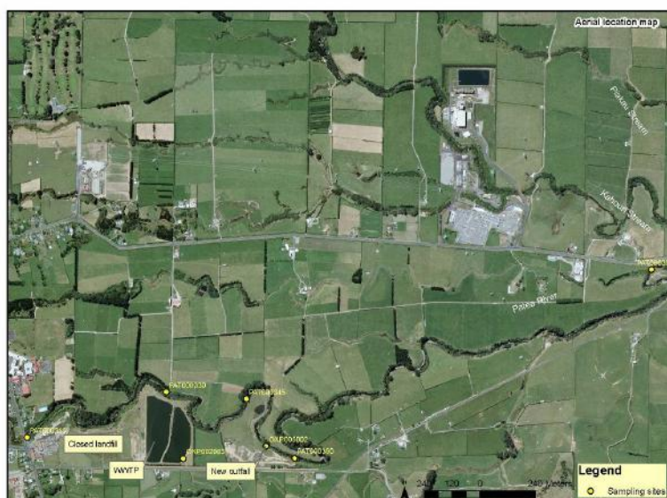
Figure 2 Aerial photo of site and location of sampling sites since the upgrade of the WWTP
