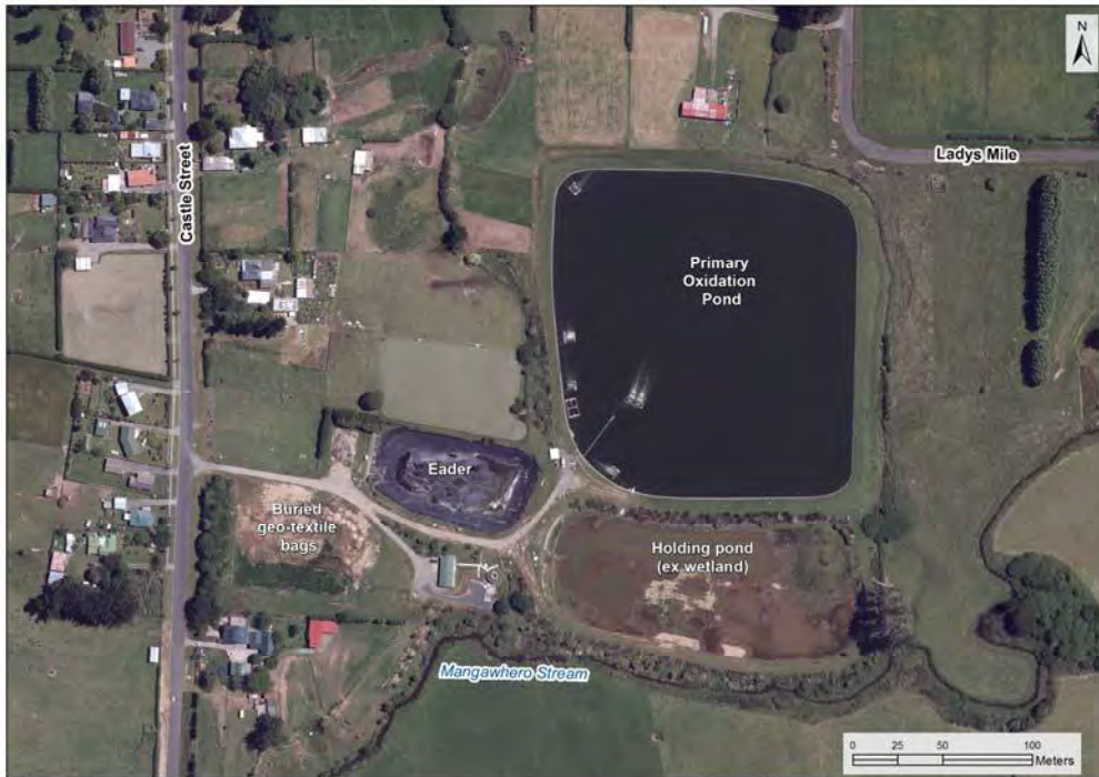
Figure 2 Aerial view of the Eltham WWTP showing the sludge geo-textile bags disposal area (lower LH corner) near the plant entrance [Note: the wetland (lower, centre) was converted to a holding pond in early 2011]
