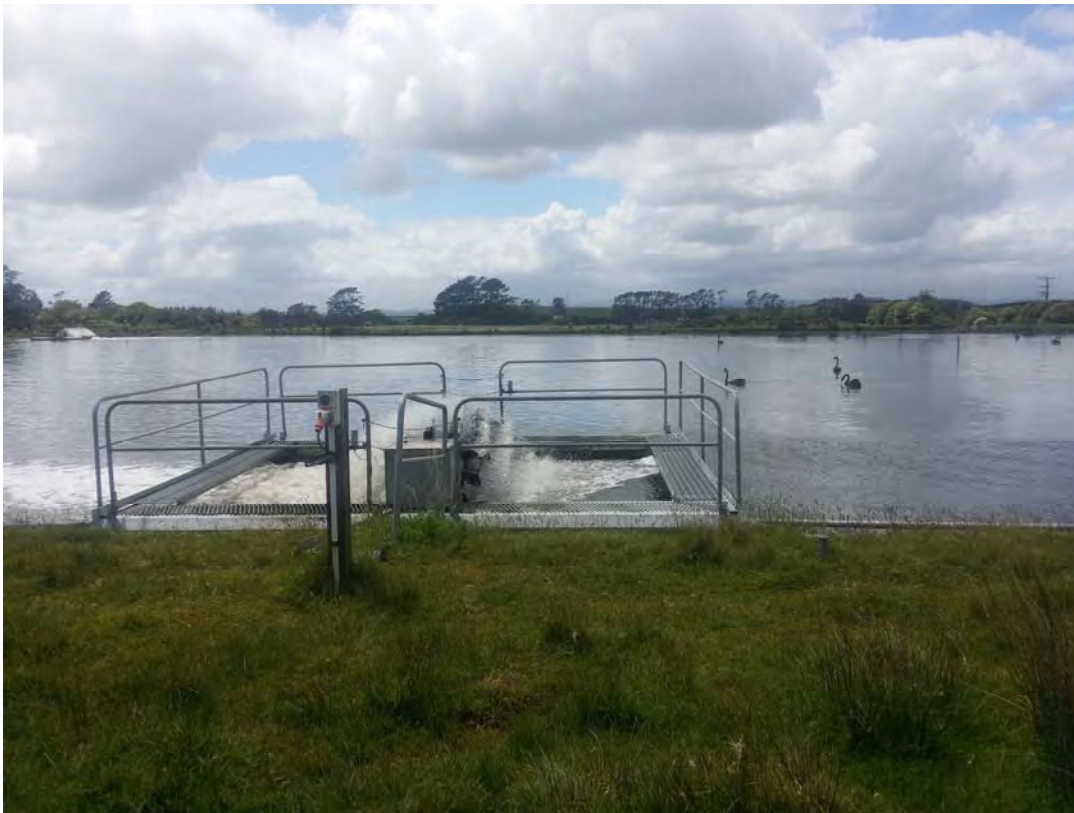
Photo 3 View of Stratford WWTP primary pond with aerators operating
