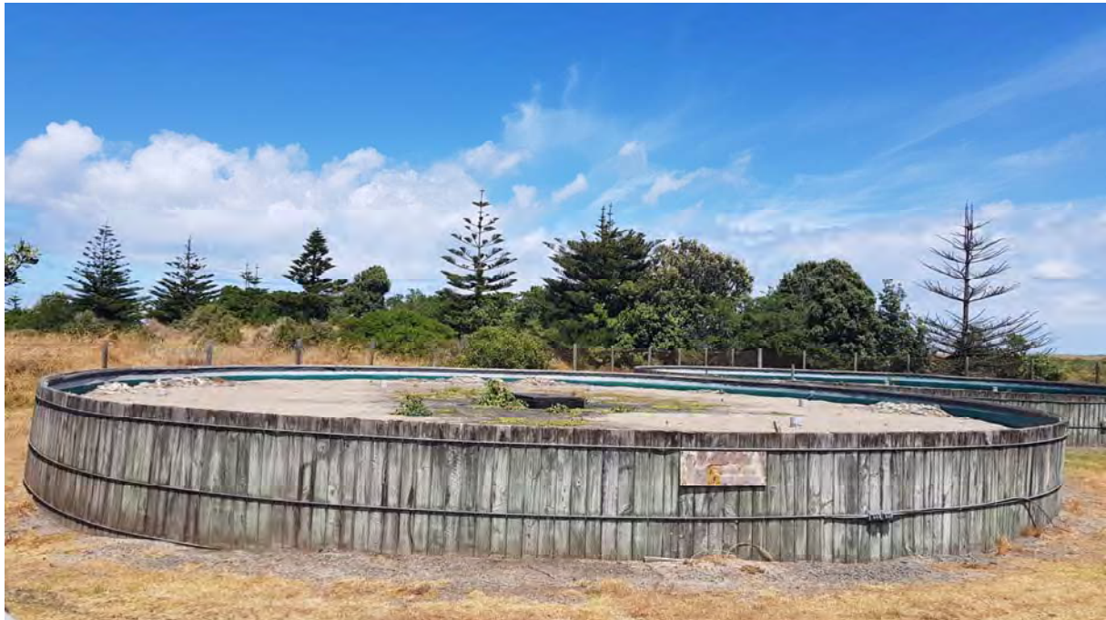
Photo 1 Low-moderate weed growth on the eastern filter bed at Wai-inu Beach Settlement (20 December 2017)
