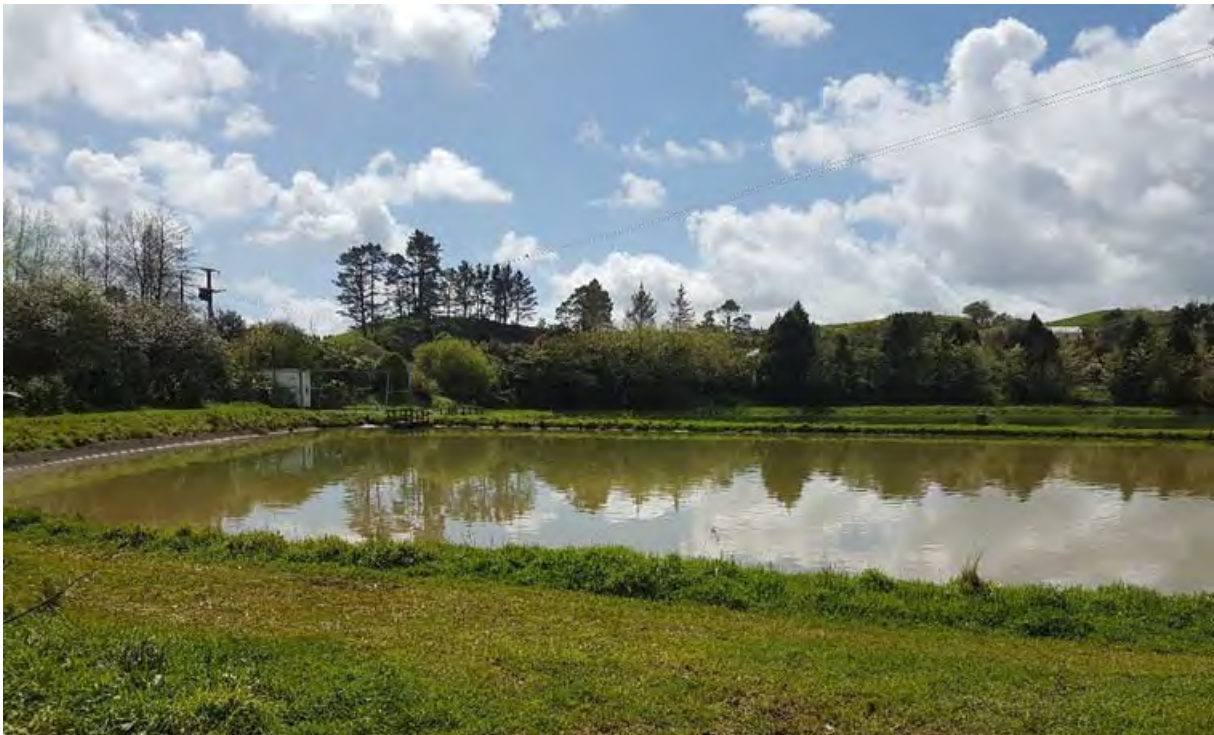
Photo 2 The Inglewood WWTP main pond
