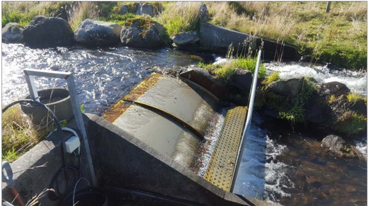
Photo 1 CCCWSL's weir and intake screen
