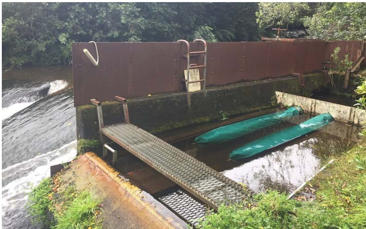
Photo 1 Inglewood contingency/farm supply intake and weir in the Ngatoro Stream
