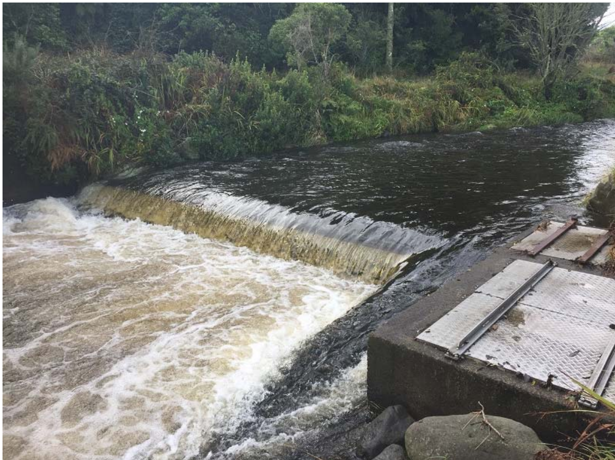
Photo 1 Okato water supply intake weir in the Mangatete Stream
