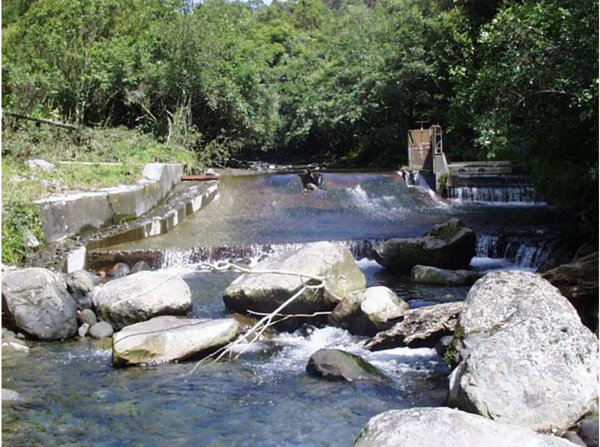
Photo 3 Ngatoro Stream weir and fish pass
