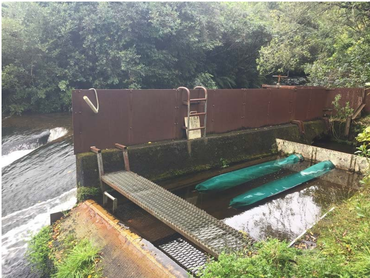
Photo 2 Inglewood contingency/farm supply intake and weir in the Ngatoro Stream
