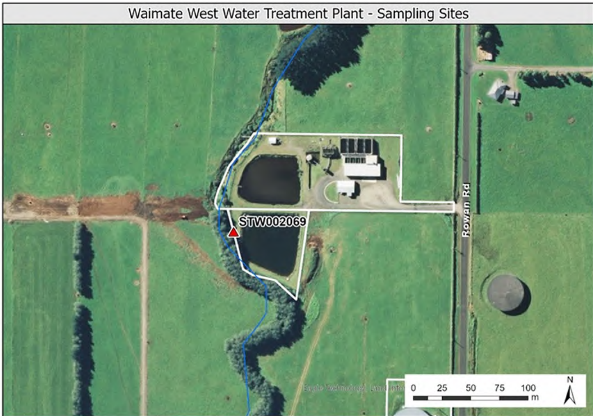
Figure 5 Aerial photo showing filter backwash sampling site for the Waimate West WTP
