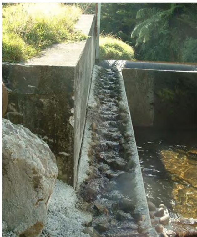
Photo 1 Fish pass on the STDC weir in the Mangawhero-iti Stream
