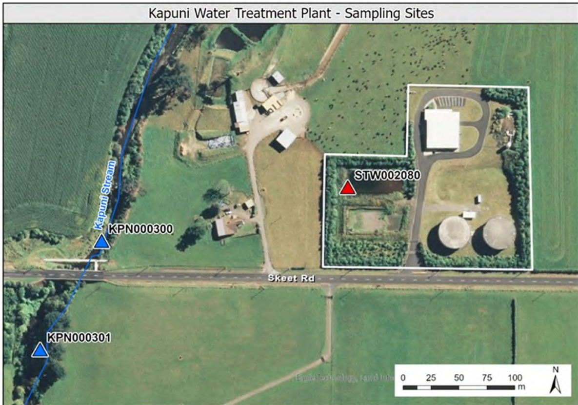
Figure 3 Aerial photo showing sampling site locations for the Kapuni WTP
