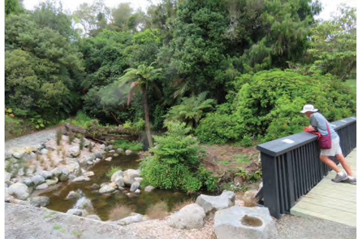
The Weka Wetland established at the site of the old ponds which are now connected by a culvert and bridge railing. The planting features divaricating native shrubs.
