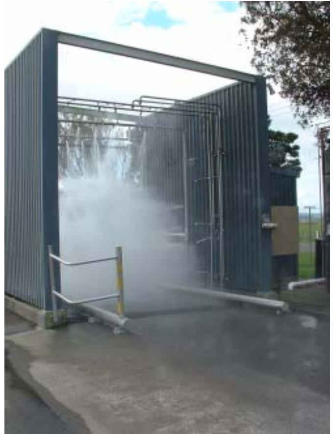
Photo 2: Purpose-built wash areas are designed to cope with large volumes of dirty water
