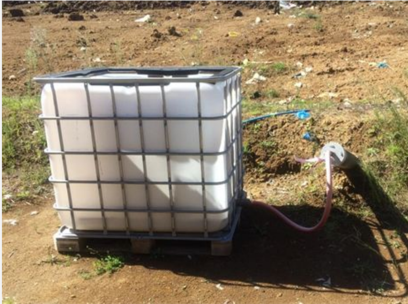
Photo 1 Trial biofilter installed on one of the protruding leachate lines
