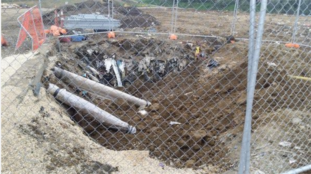
New style special waste pits – small, with cover applied soon after waste received
