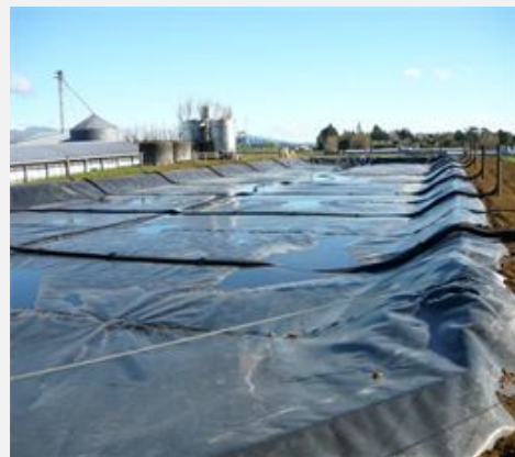
Photo 5 Covered anaerobic pond – in readiness for capturing methane gas
