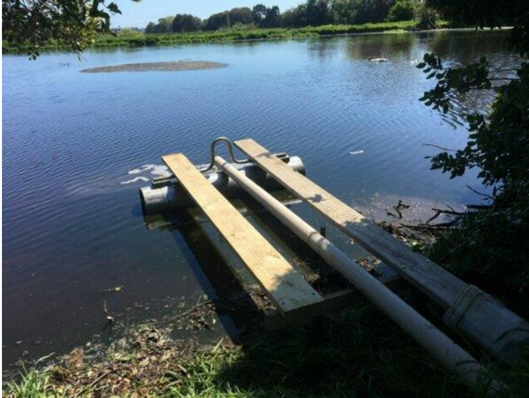
Photo 6 New pipe bridge allowing sampling of partially treated effluent from the covered digester discharging into the anaerobic pond 1
