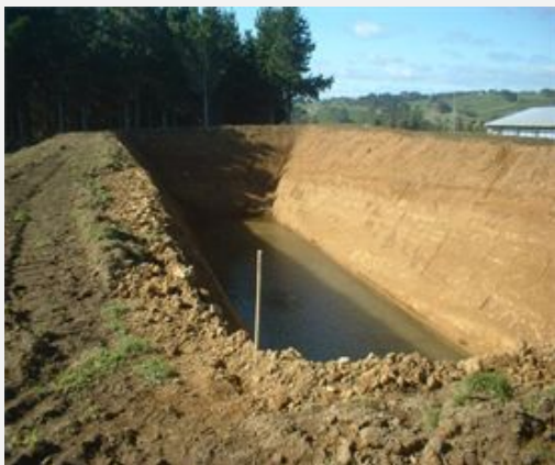
Photo 4 2008-The start of installing the covered anaerobic pond
