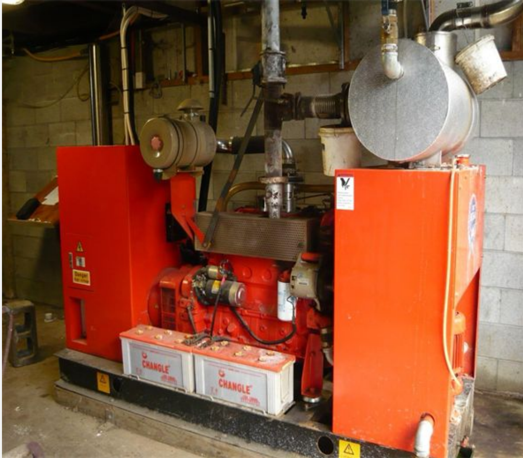
Photo 3 Generator producing 40 kw electricity for heating purposes
