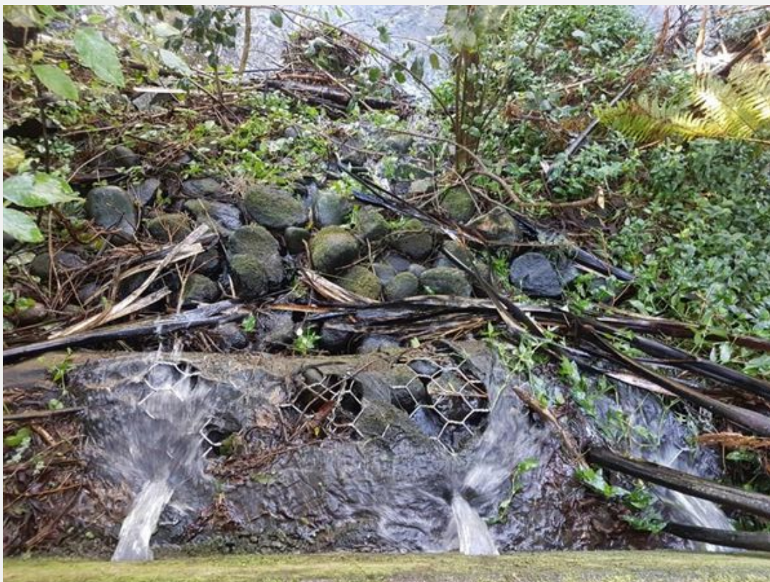
View of treated wastewater from Inglewood WWTP following heavy rain
