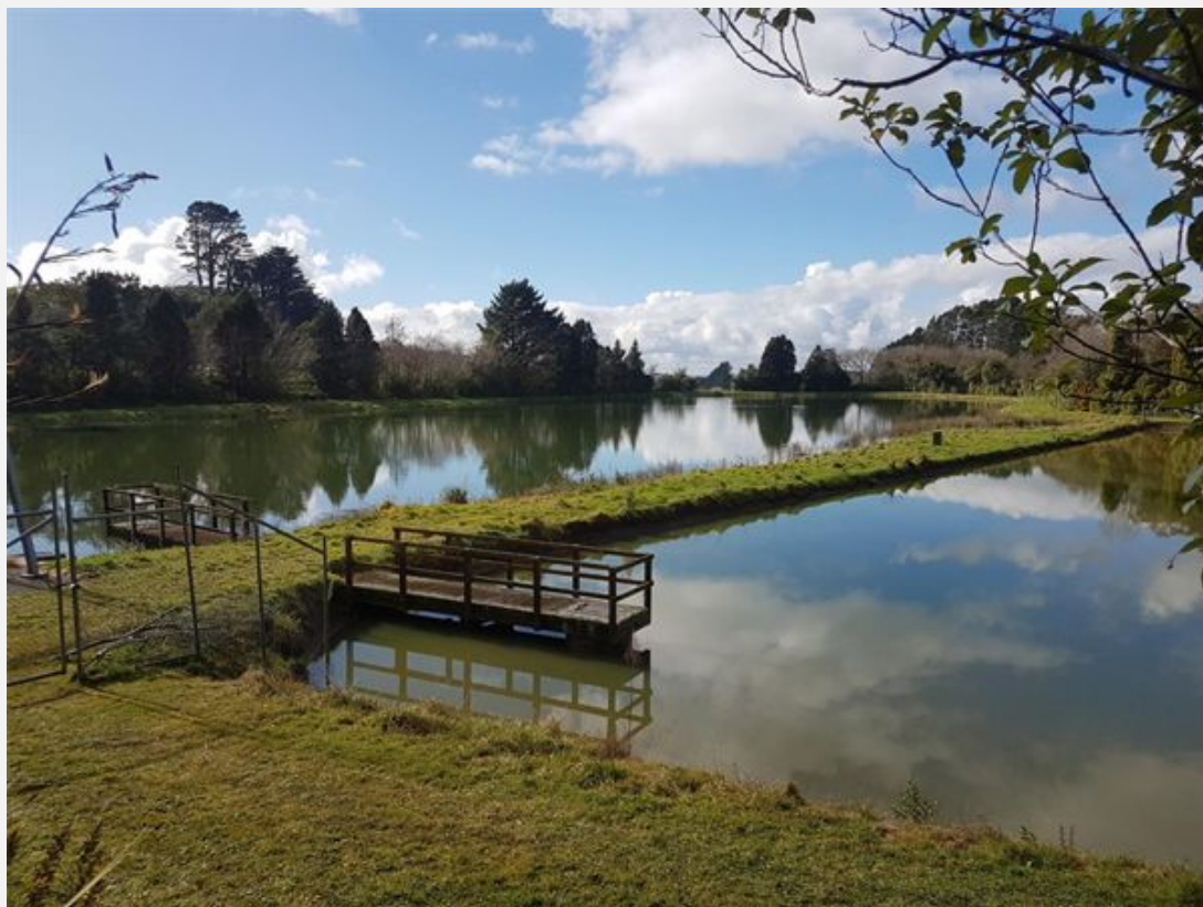
New Plymouth District Council Inglewood WWTP oxidation pond
