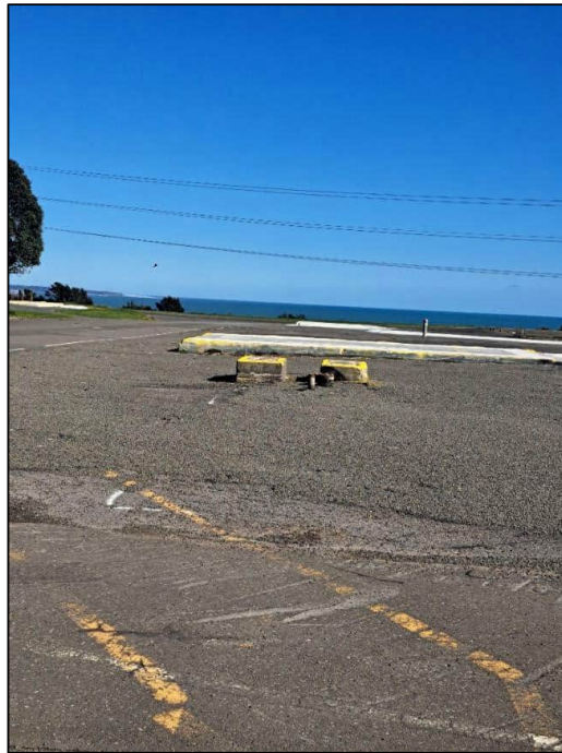
Photograph 2: Welded fill point for process water piping adjacent to Building 09.
