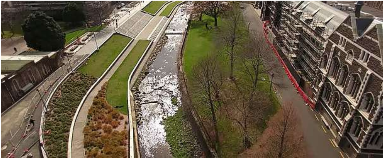
Water of Leith at University of Otago clock tower showing the amenity value achieved through sensitive design of river control and flood management works.
