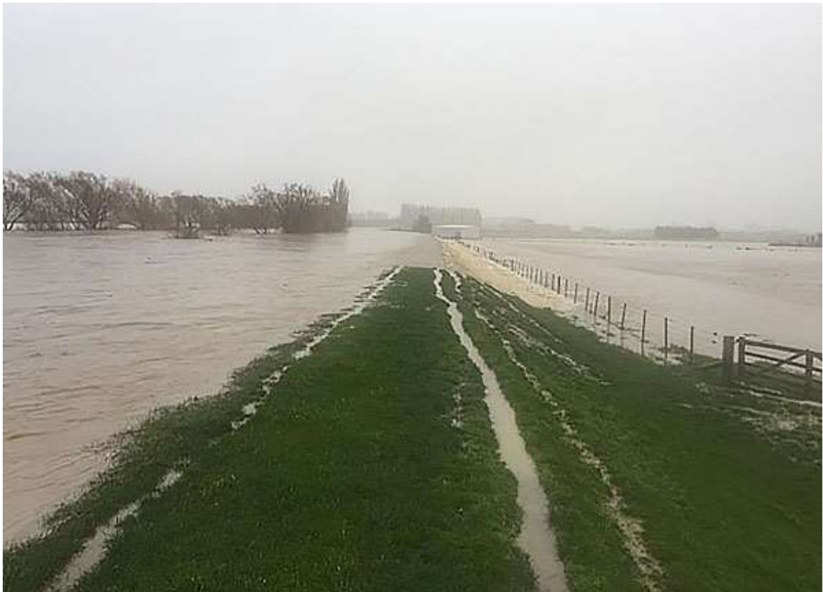
Photo: Selwyn River stop-bank overtopping in July 2017.
