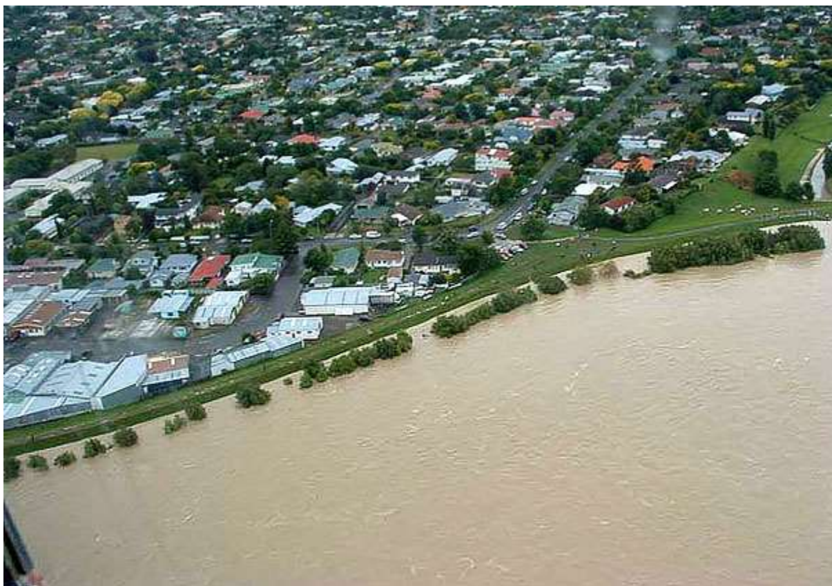
Figure 1.1: Stop-banks protected Palmerston North from inundation during the 2004 Manawatu River flood event. Source: teara.govt.nz
