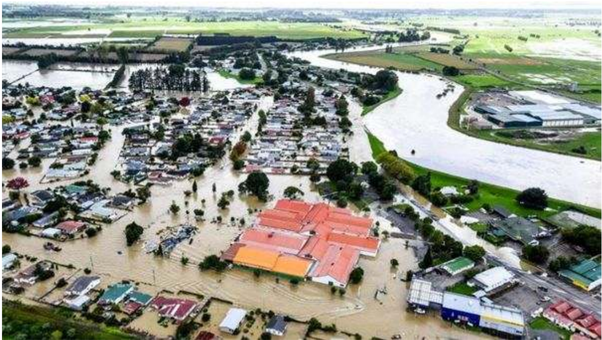
Extensive inundation of Edgcumbe following the failure of Rangitāiki River stop-banks in April 2017.
