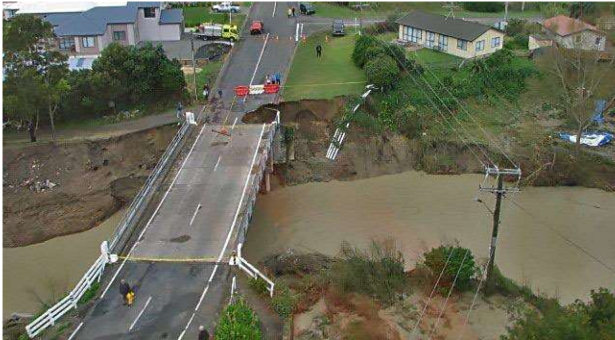
Waimarama Bridge North, Hawkes Bay Floods 2011
