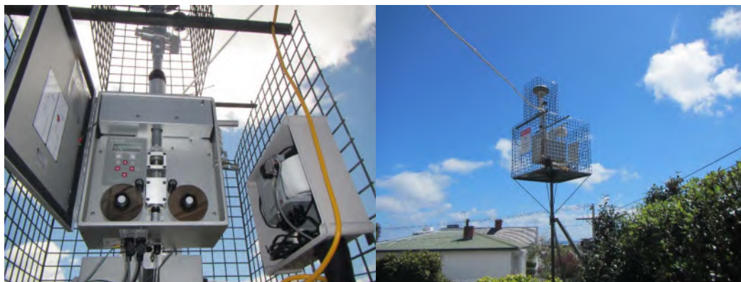
Figure 4 E-BAM set-up and installation at Central School, New Plymouth
