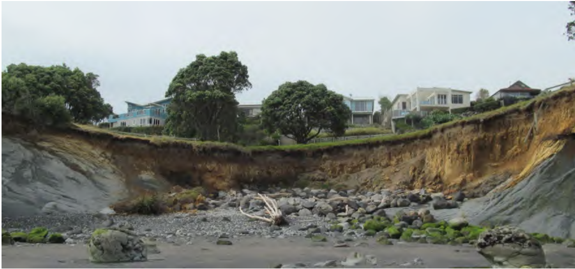
Coastal Erosion at Motukari Reserve, Onaero
