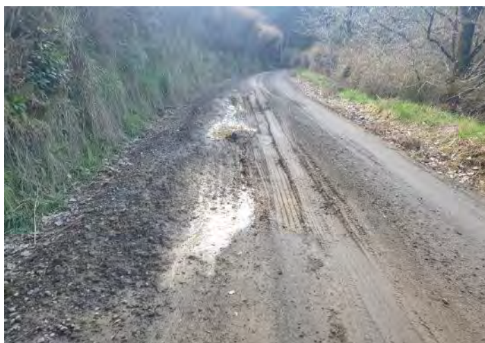
Puniwhakau Road – damage due to logging activity after 4 weeks.
