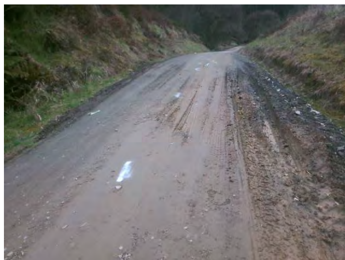
A failed area to be dug out and filled with 150mm gabion rock to strength the road foundation.
