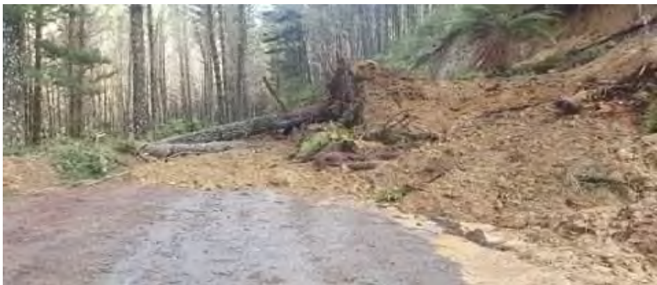
Slip including fallen trees on Mangaoapa Road - before
