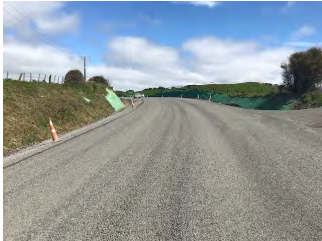
Shovel Ready Projects - Opunake Rd Safety Improvements.
