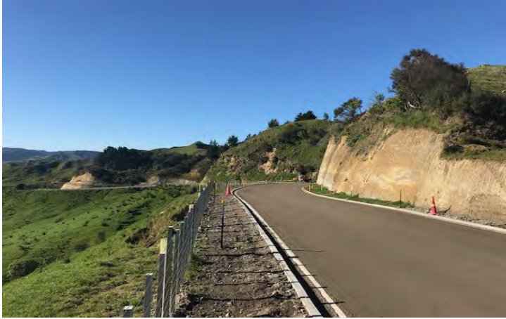
Mangaotuku Rd Improvement – from the top of the saddle looking south prior to resealing.
