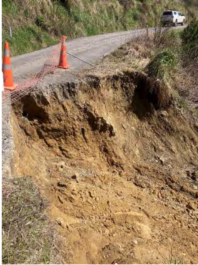
Mangare Road Slip - Before
