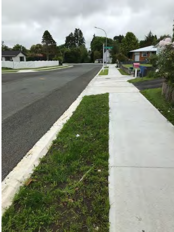
New Footpath, kerb and Channel in Montjoy St, Stratford.
