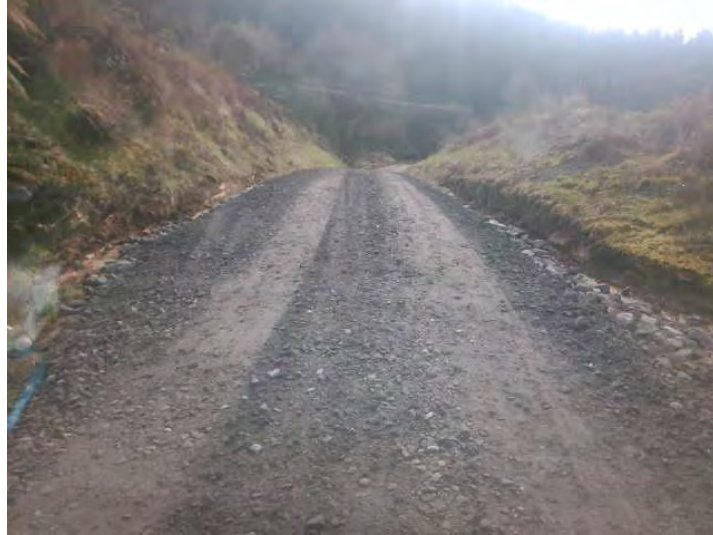
The dig-out filled with 150mm gabion rock and capped off with AP65.
