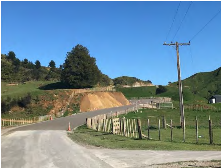
Mangaotuku Rd Improvement – from the valley floor looking north
