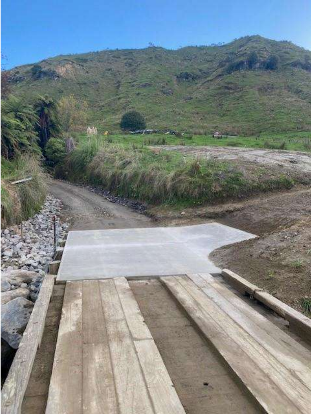
Figure 4 – Completed repairs to the eastern abutment of the bridge.
