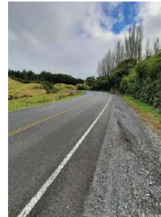
SH4 RDC WDC Boundary renewal
