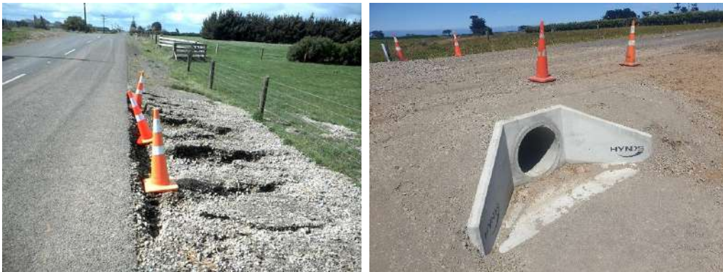
Tempsky Road – Culvert replacement – Before and after photo
