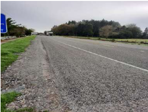
SH3 Inglewood South rehab
