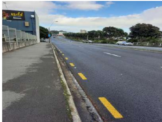
SH44 Egmont to Liardet Structural Asphalt and thin asphalt
