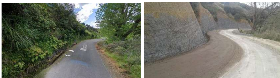
- Morea Road – sight benching widening- Before and after photo.
