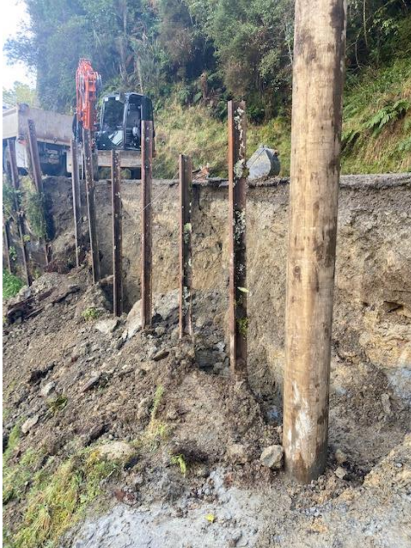
Figure 2 – Repairs to the railway iron retaining wall on Mohakau Rd
