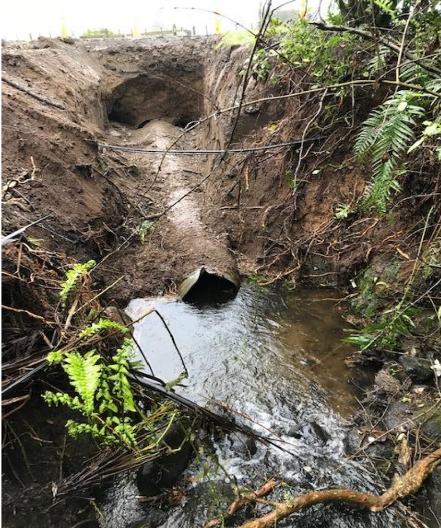
Figure 5 – The roof of the cavity removed exposing the steel culvert
