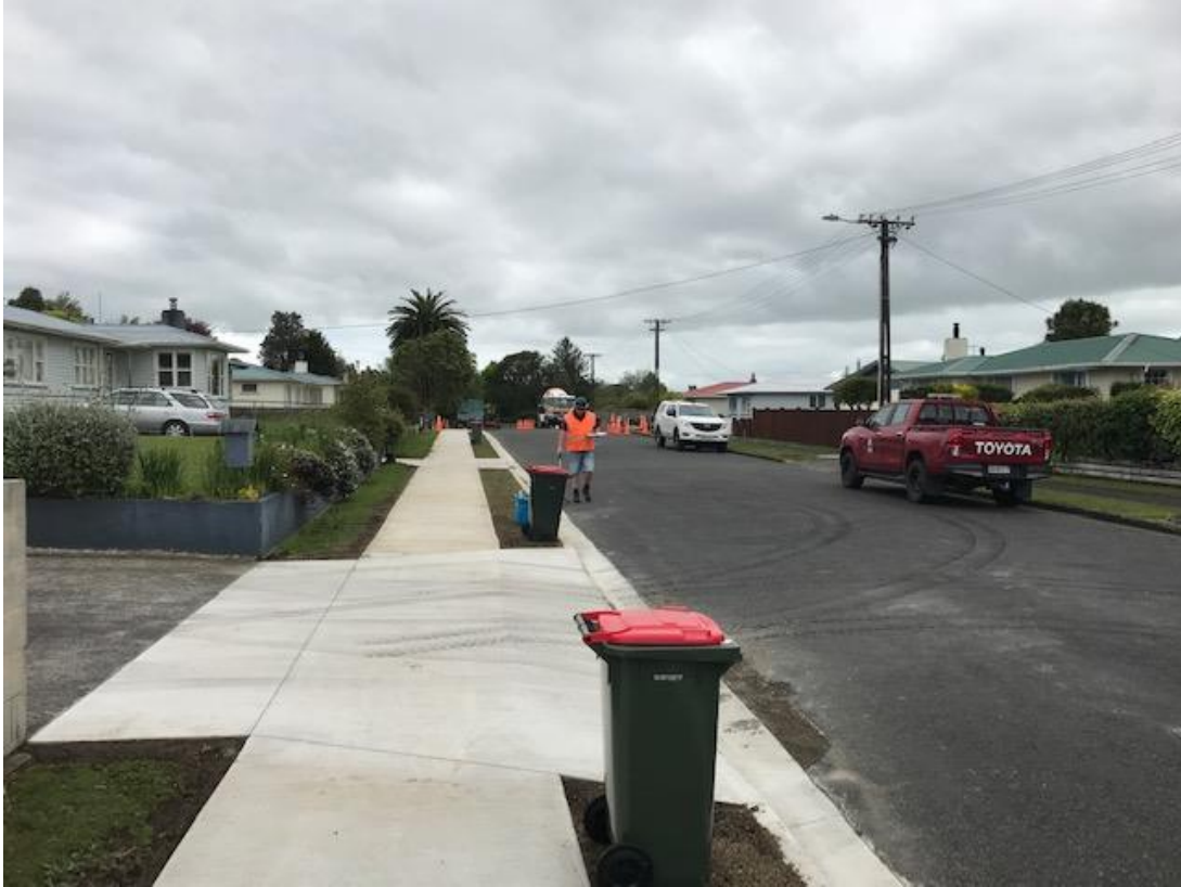
Figure 1 – Replacement of kerb, channel and footpath in Fabian Street.
