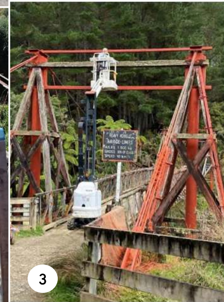
3. Goldseal being applied to the bridge.
