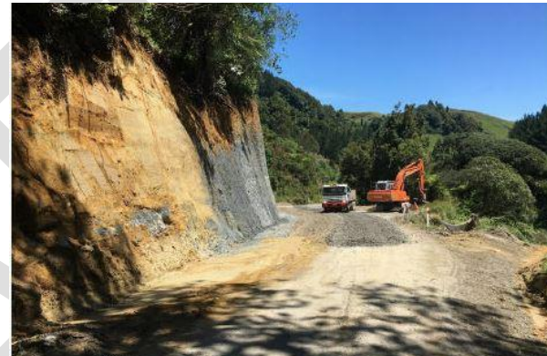
Mangaoapa Road – bank trimming and road strengthening for logging operations.
