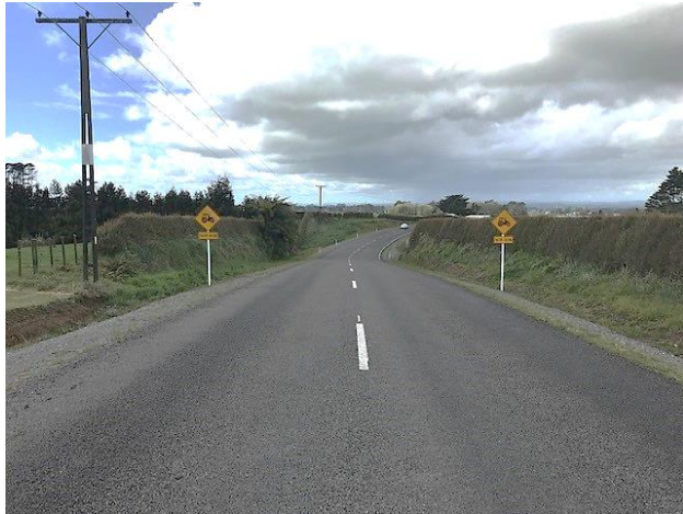
Monmouth Road pavement rehabilitation
