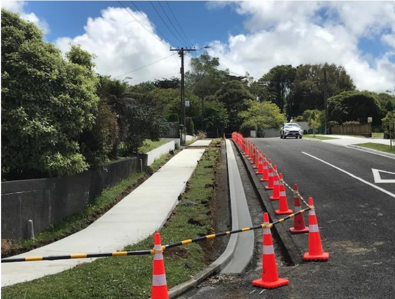
Figure 7 – Footpath, Kerb and Channel replacement in Lysander Street.
