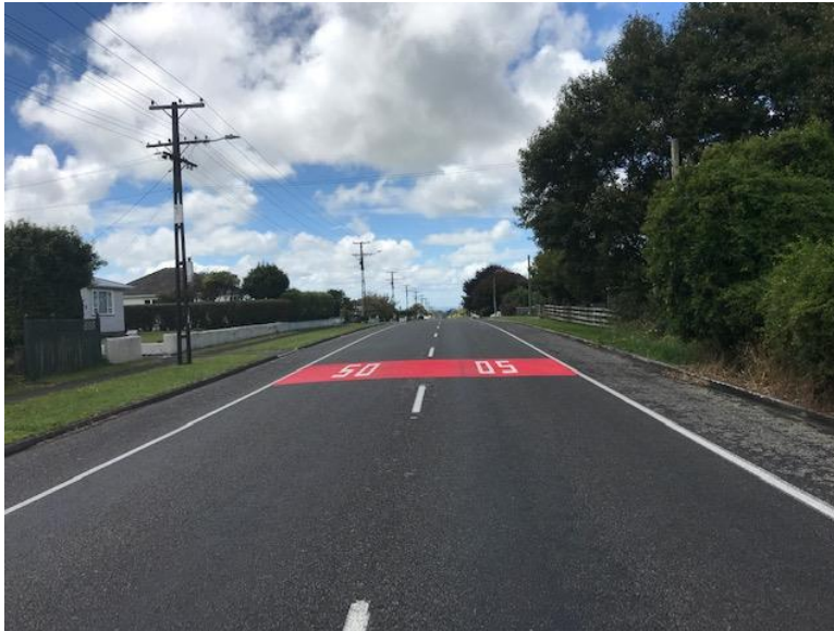
Figure 8 – Red “threshold” markings to highlight the speed limit on Celia Street
