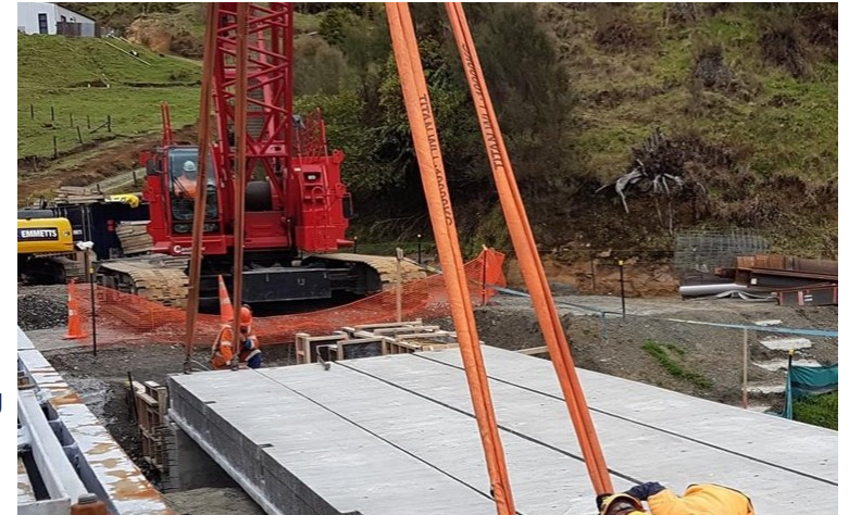
Bridge during construction
